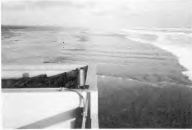
Photo. 2 Maximum wave run-down ( taken from the rooftop of HORF ).
