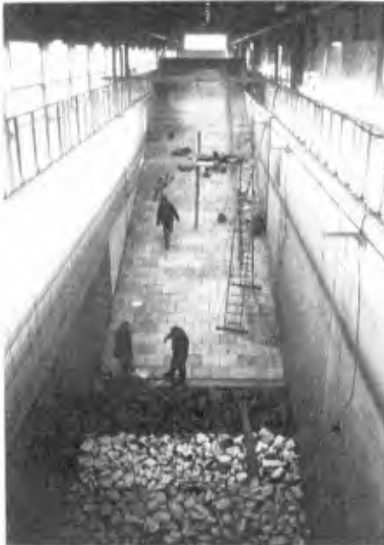
Figure 2. 1 to 4 Sloping Dyke Revetment in the Large Wave Channel
