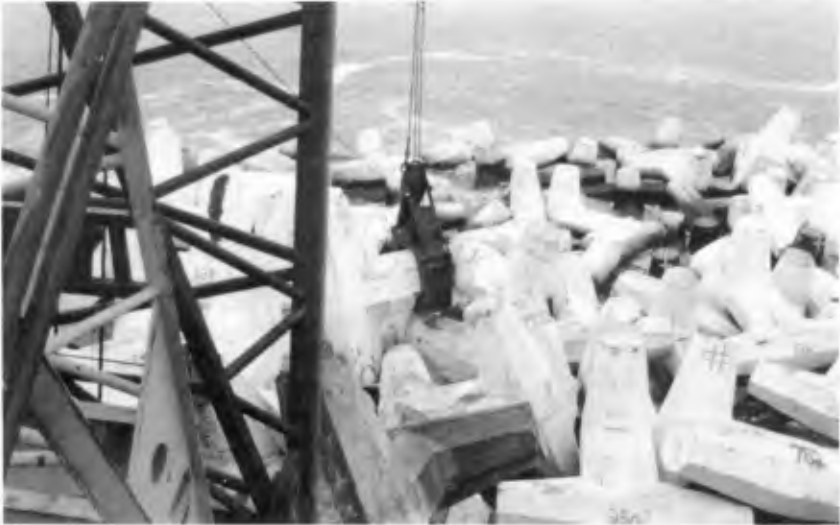
Figure 1: 38-tonne Dolosse at Crescent City, CA
