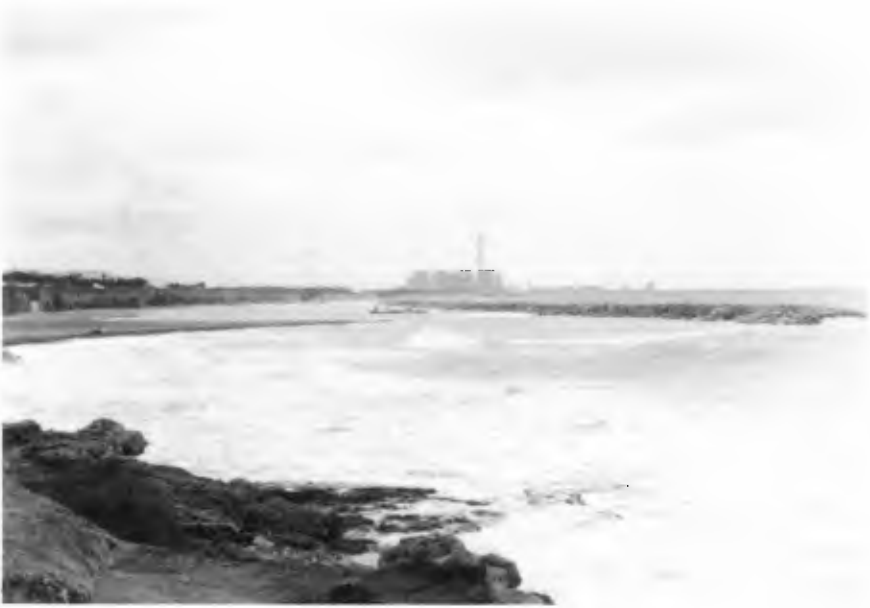
Fig.7. The first from the south of detached breakwaters and the tombolo
