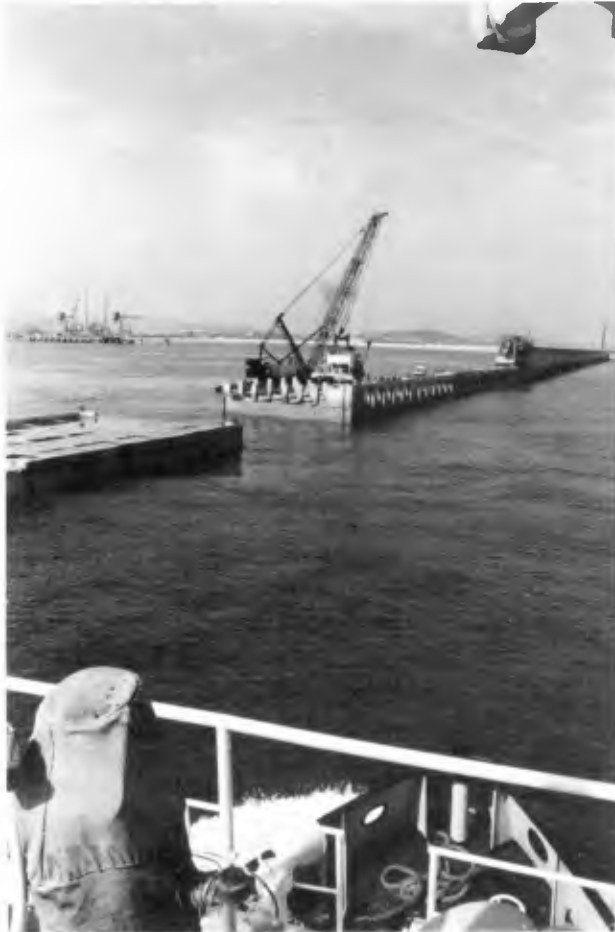
Perforated Caisson Breakwater at Porto Torres, Sardinia
