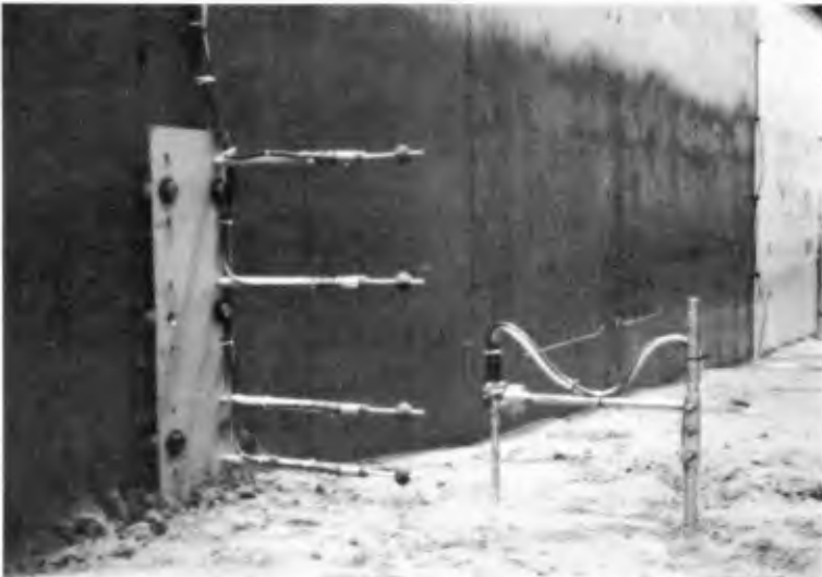
Fig. 4. Vertical arrays of current meters and optical backscatter sensors
