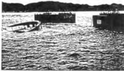
Photo. 1 Slid Caisson in Sakai Port
