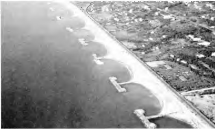
“T” Groins and Nourishment Protecting Coastal Railway
