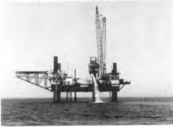
FRP RISER PIPES MADE UP INTO 120' STRINGS CAN BE SEEN ON THE RIGHT SIDE OF THE JACK- UP RIG
