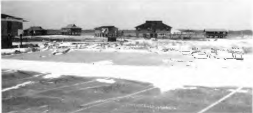
Photo 1. Typical buildings elevated to meet construction standards. Note foundation of demolished building in foreground.
