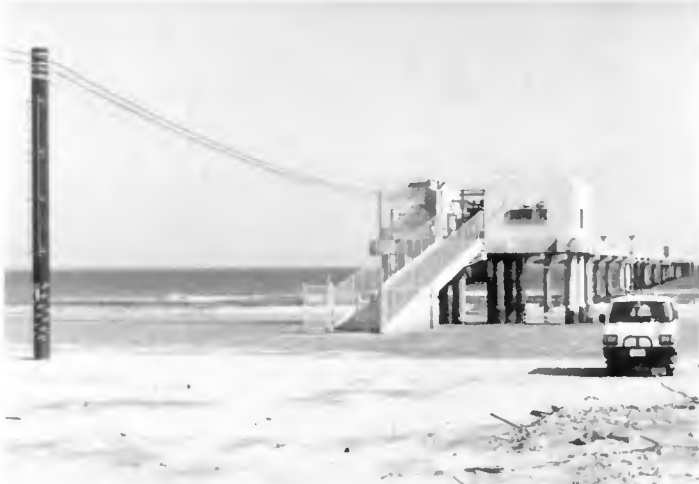
Photo. 1 Side view of HOLF ( in a calm condition )
