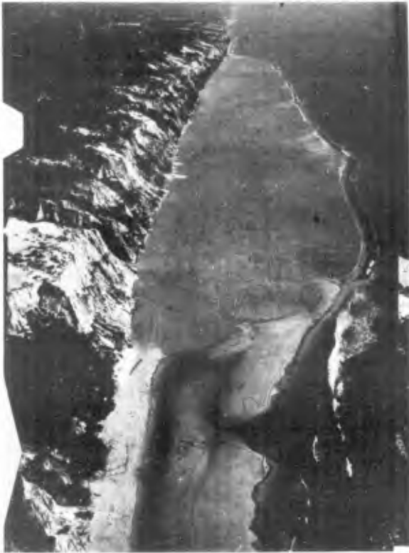
Fig.5.- Aerial View of the Protruding Area
