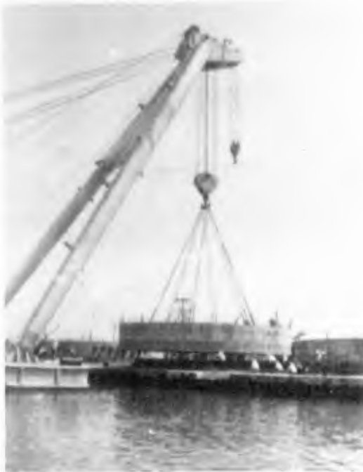
Fig. 5. Cylindrical caisson fabricated on quay apron.
