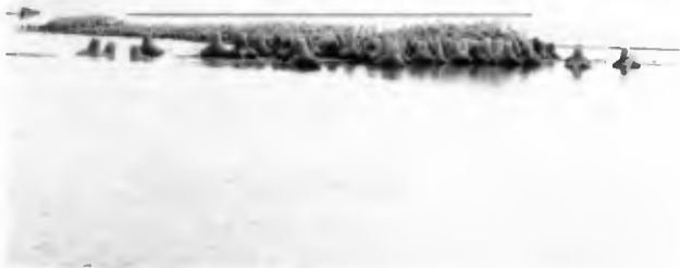
(a) perspective scene of damaged breakwater
