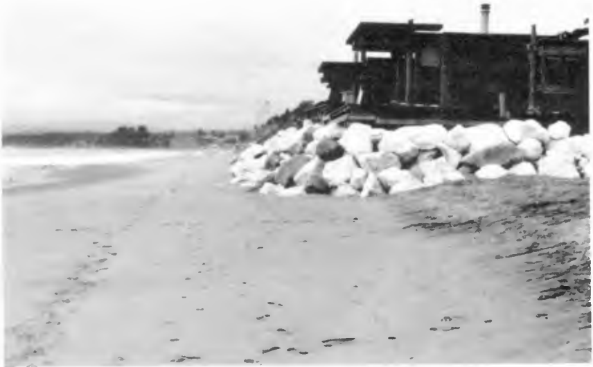
Figure 7. Early winter conditions. Berm has retreated behind revetment leaving uniform planar beach in front of revetment and control beach.
