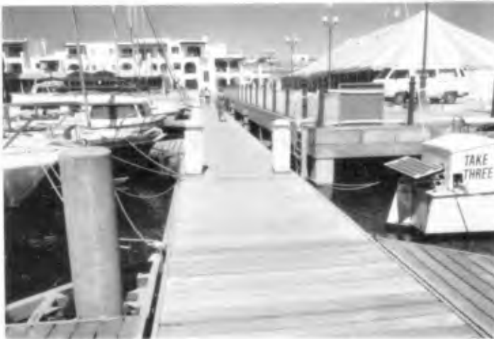
FIGURE 16 : REVTMENT, BOARDWALK AND FLOATING WALKWAY
