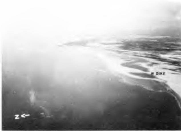
Figure 13. West Dike (10 Months After Closure) Date: 01/25/89 Hour: 13:50 W.L.= + 1.1m
