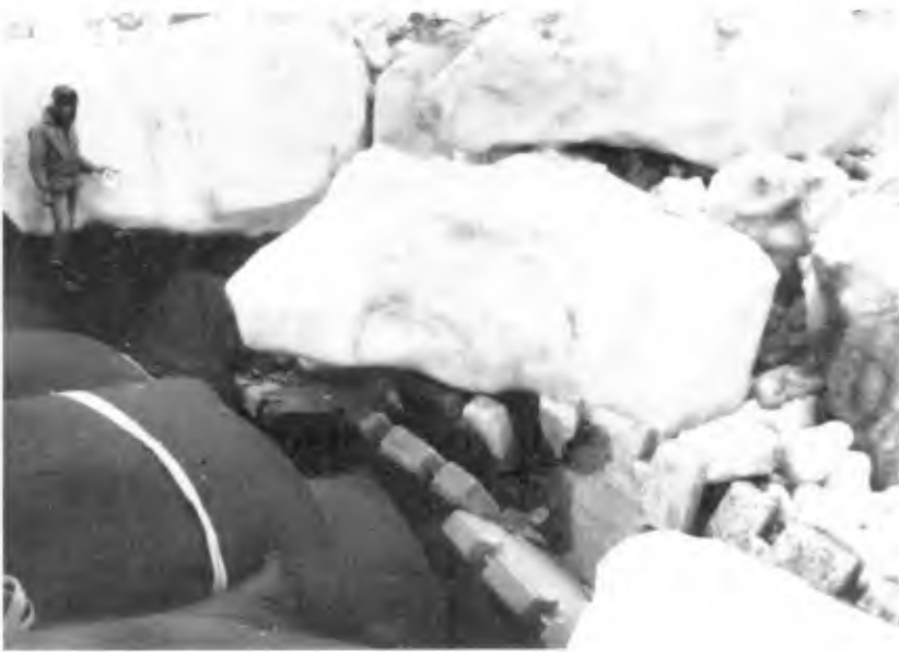
PHOTO 5: BLOCK DISPLACEMENT BY LARGE ICE IMPACT, AUGUST 1988
