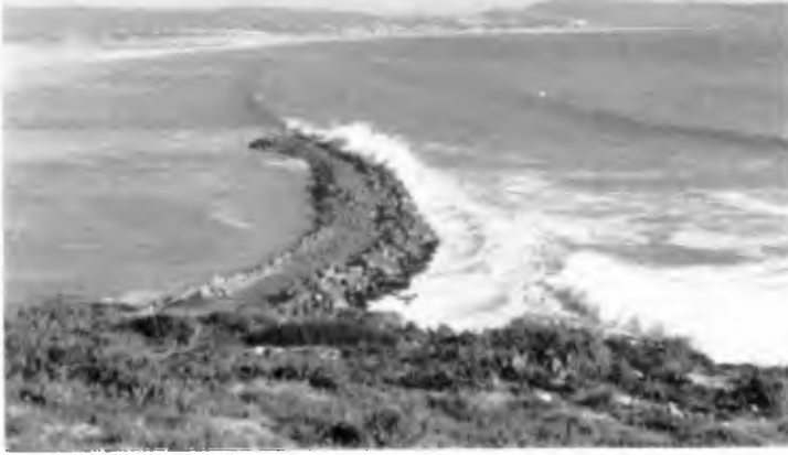
FIGURE 9 : BREAKING WAVES ON MAIN BREAKWATER DURING CONSTRUCTION
