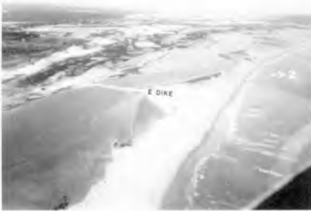
Figure 11. East Dike (Closer View) Date: 04/07/88 Hour: 14:23 W.L. = +0.8m
