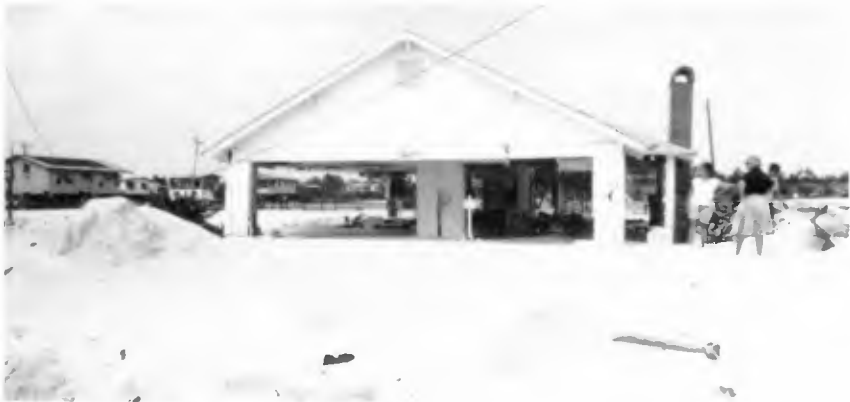
Photo 3. Wave damage to "old" building in the overwash zone. Originally and presently an A-zone, but a V-zone in 1980-1.
