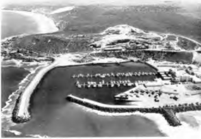
FIGURE 11 : COMPLETED HARBOUR WITH MAIN BREAKWATER ON LEFT SIDE
