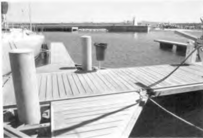
FIGURE 17 : FLOATING JETTY SYSTEM
