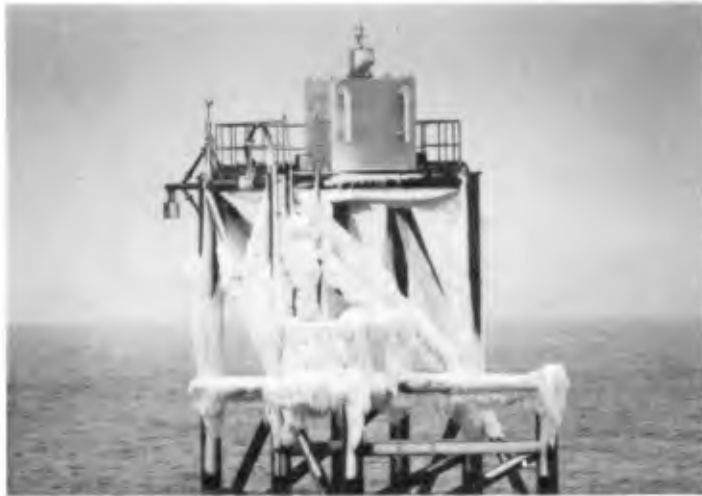
Phot.1 Offshore experimental structure
