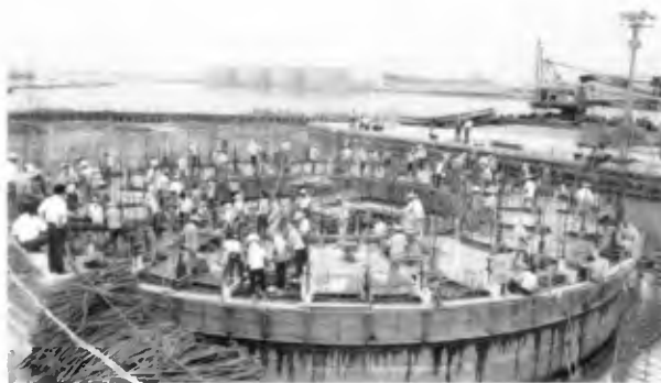
Fig. 4. Cylindrical caisson fabricated inside the dock.
