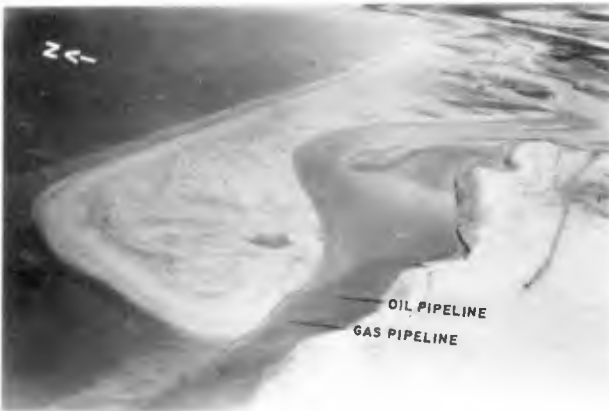
Figure 6. Undermined Pipelines Date: 03/02/88 Hour: 10:24 W.L.= +0.7m
