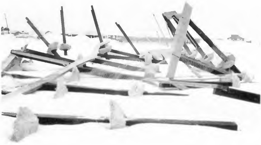
Photo 2. Undermined foundation of "new" building in erosion zone.
