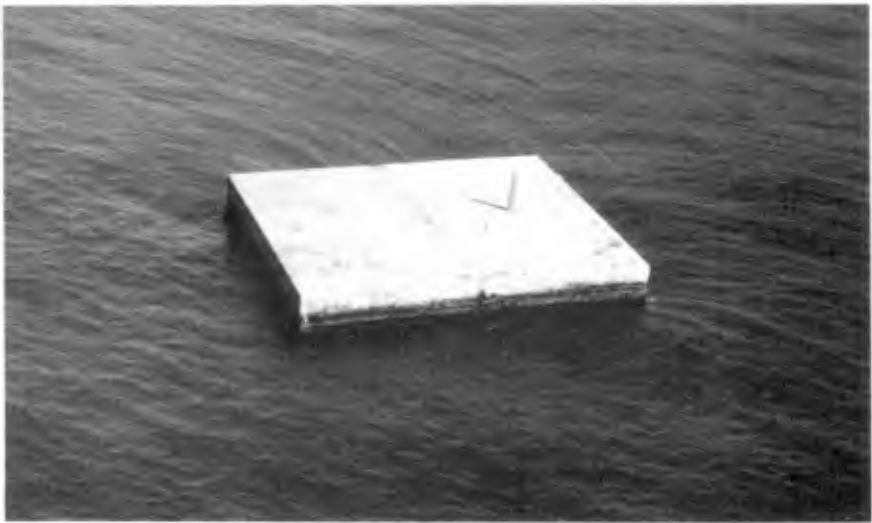
Fig. 10 Test breakwater at Tomakomai Port
