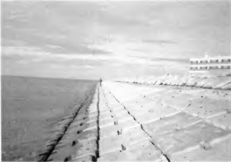
Plate 3. Concrete Mat Armor on the Endicott Project
