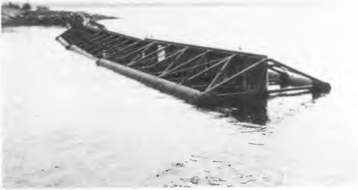
Fig. 4. The A-frame breakwater at Lund (removed in 1987).
