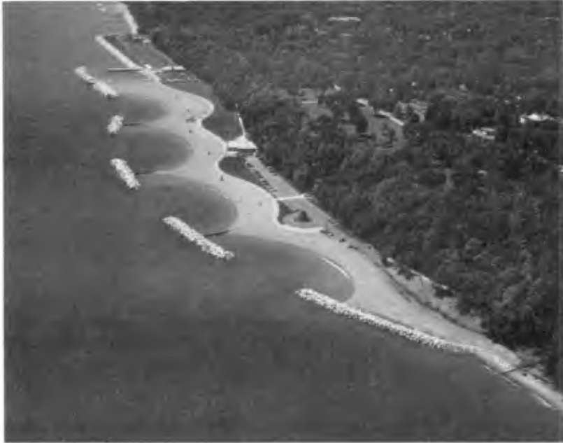
Figure 3 COMPLETED FOREST PARK PROJECT
