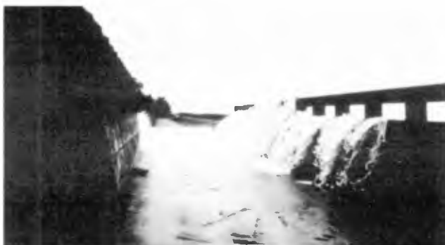
Photo 14. Heavy waves attacked the Kurobe Coast, and some of them overtopped the experimental seawalls.
