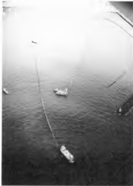
Figure 9. Connecting Pipe Sections 1A and 1B, Kawaihae Harbor
