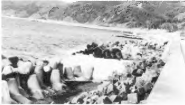
Photo 4. Before the experimental works on Hongo Coast.
