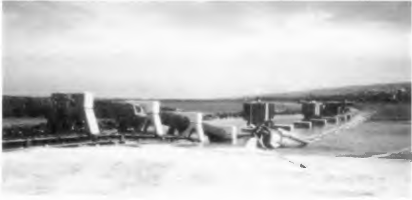
Figure 8. Pipe Haul, Kawaihae Harbor
