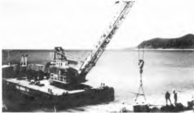
Photo 5. The experimental seawall under construction.
