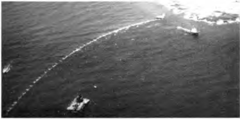
Figure 10. Aligning Pipe Section 1, Keahole Point
