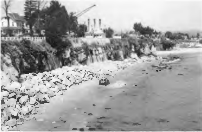
Figure 6 - Seawall during Construction (April 1962)
