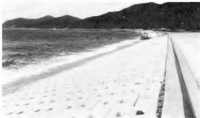
Photo 6. The experimental seawall completed.
