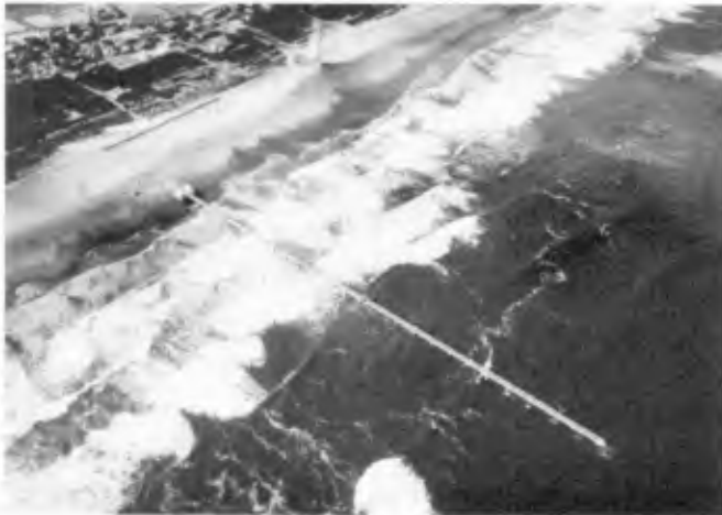
Photo. 1 Hazaki Oceanographical Research Facility
