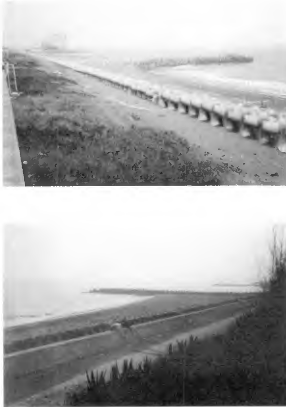
Fig. 13. Field results of shore protection of Kaohsiung Harbor outer breakwater
