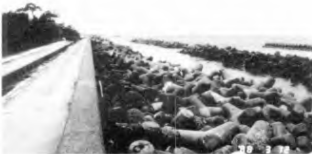
Photo 7. Left-hand side view of the experimental works.
