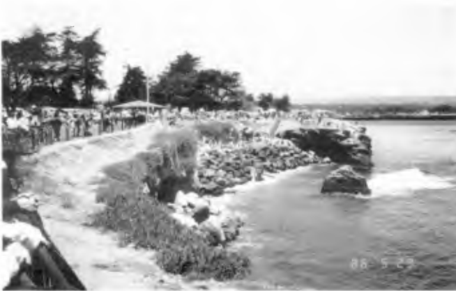
Figure 8 - Seawall near Santa Cruz (May 1988)
