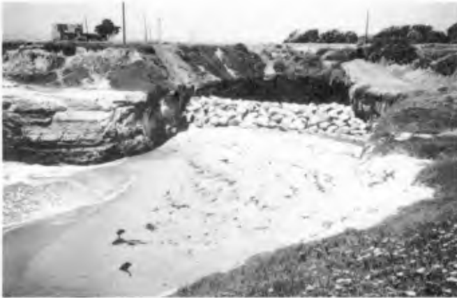
Figure 7 - Seawall Construction (May 1961)
