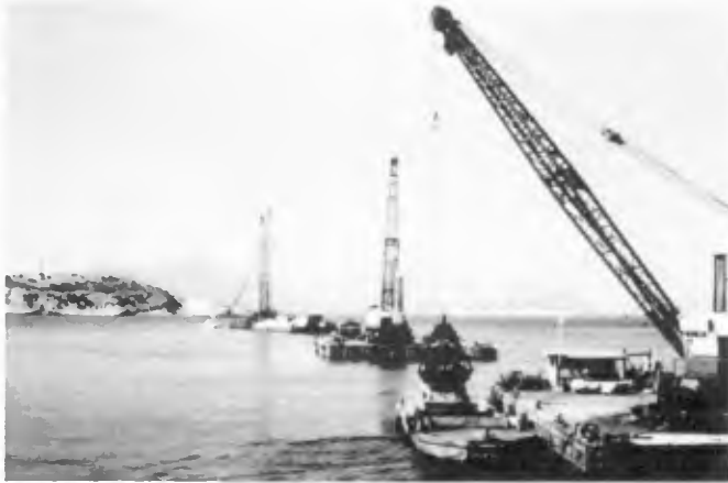
PIPE TRENCH EXCAVATION
