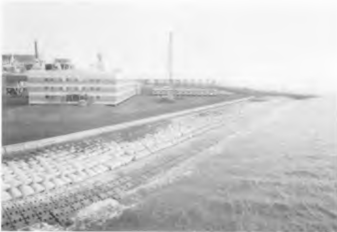
Plate 4. Articulated Concrete Mat on the Endicott Project
