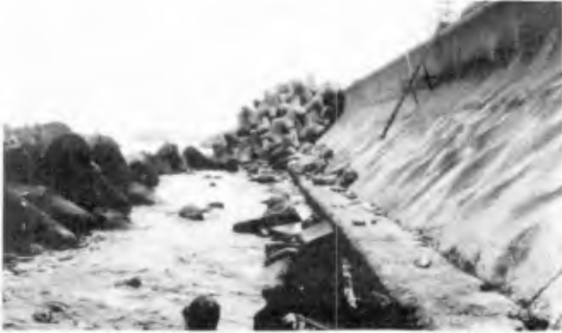
Photo 8. First, mound of armour units were removed.
