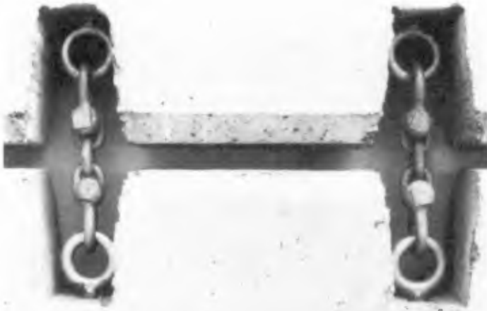
Plate 2. Chain-and-Shackle Linkage System
