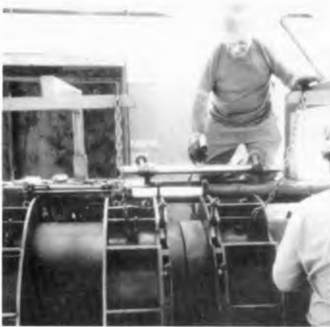
Figure 4. Polyethylene Pipe Thermal Butt Welding
