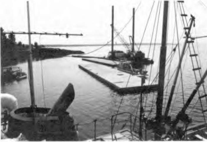
Fig. 2. The new caisson breakwater at Lund during installation.
