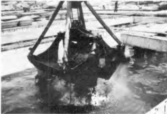
Figure 7 Asphalt Placement With Four Cubic Yard Bucket
