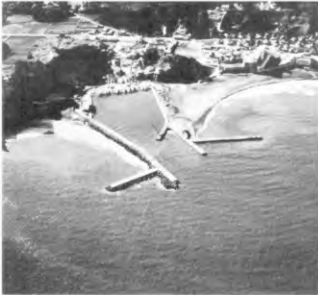
Fig. 5 Recovered Taito Harbor after rip current barrier construction.
