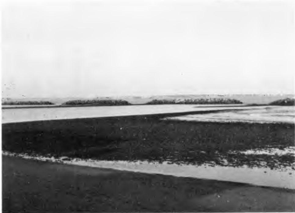
Five Sisters Breakwater showing accretion behind, Wentthrop Beach, MA
