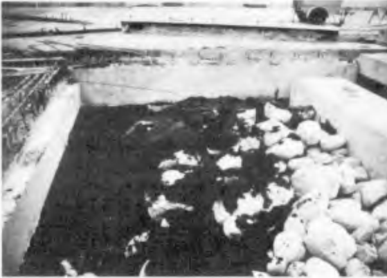
Figure 8 Asphalt Grout Partially in Place Near the Crest
