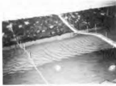
Fig. 15 An example of seabed scour near the tip of breakwater.
