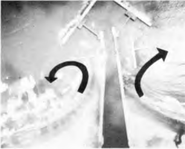
Fig. 16 Rip current barriers at Katagai Fishery Harbor. Arrows show measured rip currents.
