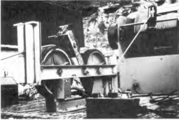
Figure 12 Pinch Wheel Distance Counter and Winch System
