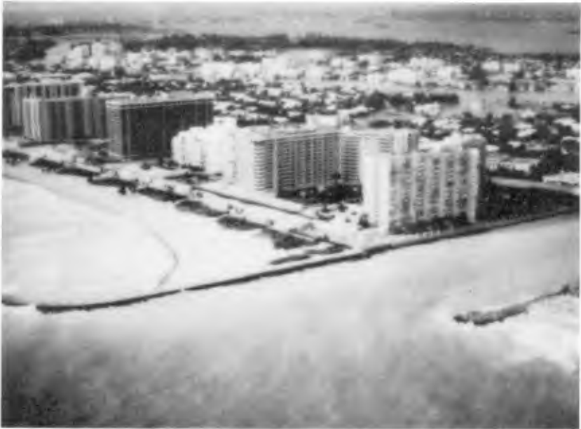
Figure 8. Beach fill at Bakers Haulover Inlet.
