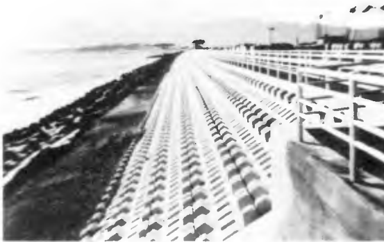
Photo.3 Restoration works completed (1978)
