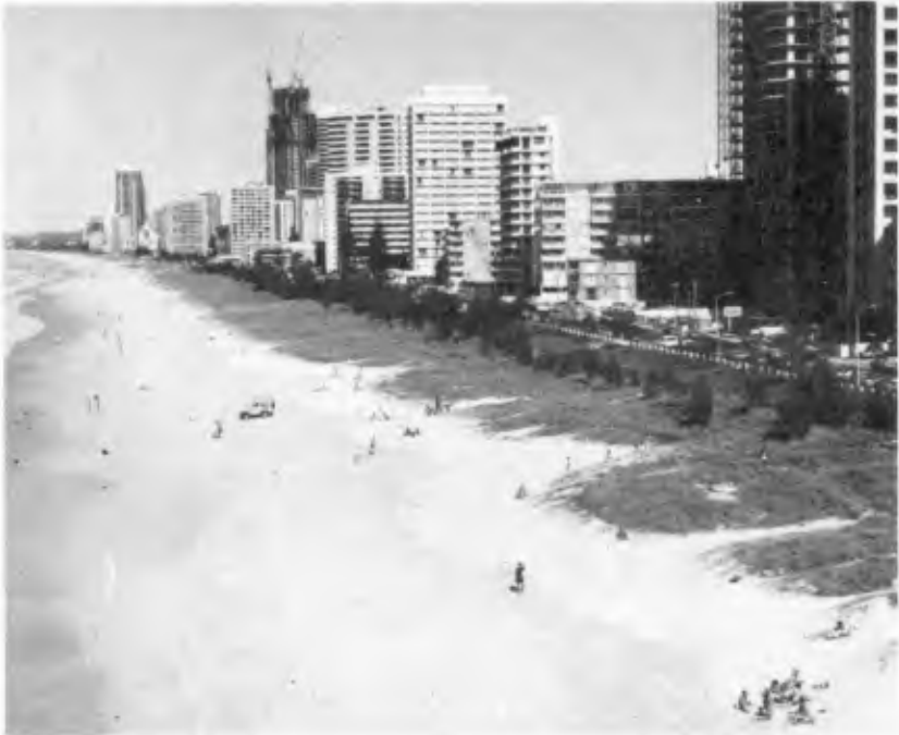
Beach nourishment to Surfers Paradise in 1974 has established a new beach and dune system in front of the seawall. The photo shows the beach in 1983 in good condition.
