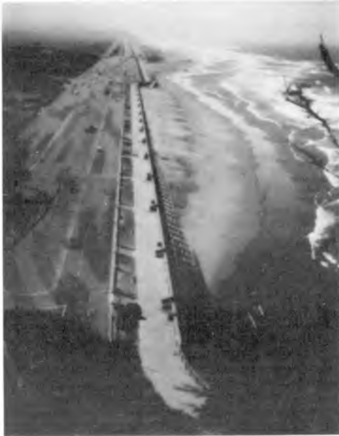
Figure 4. O'Shaughnessy seawall at Ocean Beach Esplanade, San Francisco, California.
