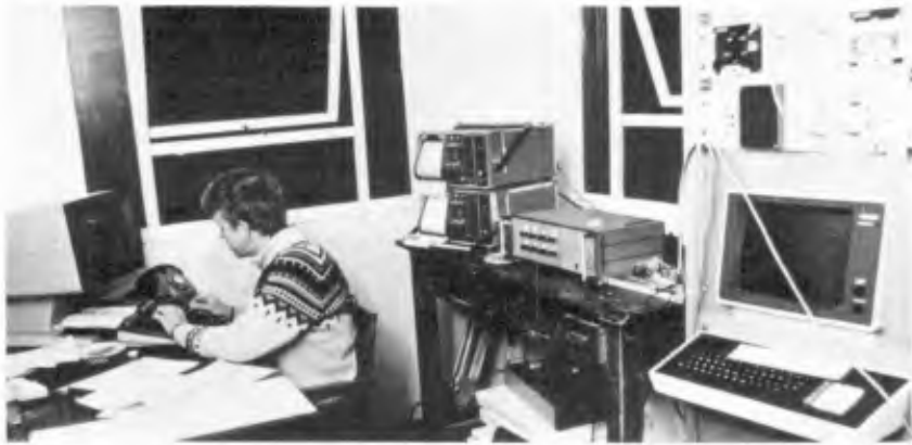
Figure 9. Data acquisition system in the control room
