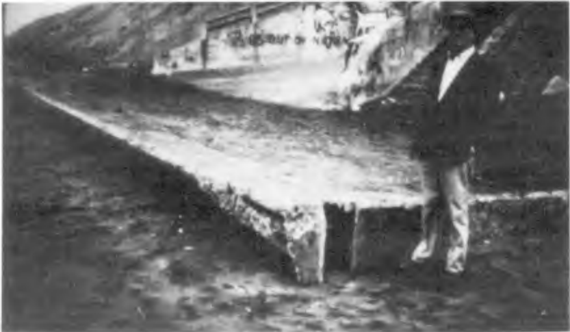
Figure 3. Taraval seawall at the South end of Ocean Beach, San Francisco.
