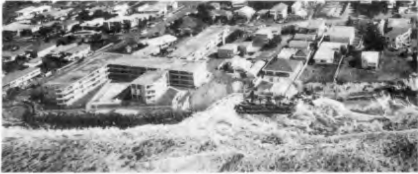
All of the Gold Coast beaches were substantially eroded by cyclones in 1967. Severe problems were experienced where development was located close to the beaches, such as in the Surfers Paradise area (pictured).
