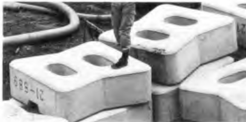
Photo.5 Lotus-Uni block ( Model 50H, 2 ton)
