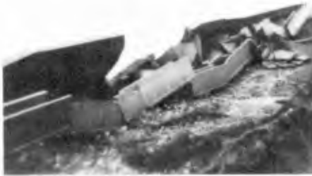
Photo.2 Vertical type seawalls collapsed
