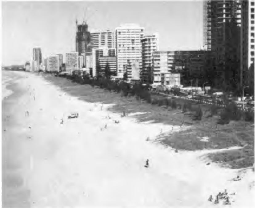
Beach nourishment to Surfers Paradise in 1974 has established a new beach and dune system in front of the seawall. The photo shows the beach in 1983 in good condition.
