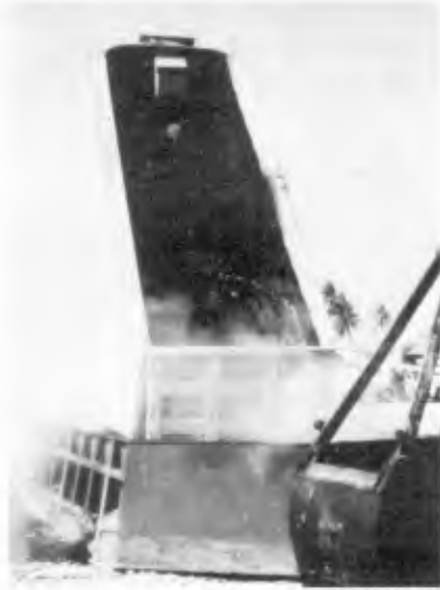
Figure 6 Asphalt Being Dumped into Rock Bin at the Site
