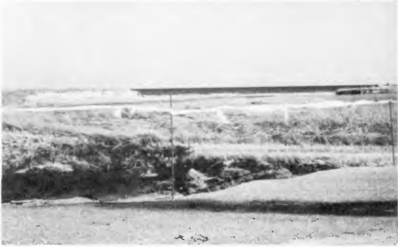
Figure 5. Gulfward view of Follets Island cut showing erosion of dunes behind beach. Highway pavement is in foreground.
