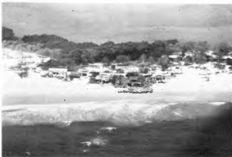
PLATE 2: - DAMAGE FROM NATURAL LONG TERM EROSION
