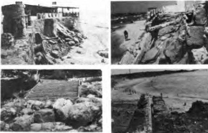
Fig. 15. Severe beach erosion near offshore structures. Fig. 15a. Heavy destruction on the beaches south of Tel Baruch structure (16/6/80). Fig. 15b. Shore buildings north of the Gaza Harbour groins have suffered heavy damage. Small nearshore structures parallel to the beach were erected here to prevent further collapses. Fig. 15c. Exposed beach basement at Bat Yam, after a severe storm (19/4/71). Damage was greater here because marine construction on a half closed pool in shallow water caused buildup of water during storms. Fig. 15d. Small bay north of King Herod's ancient harbour in Caesarea. While in operation this now submerged harbour caused heavy damage to the Roman aquaduct and therefore measures should have been taken to protect the aquaduct whose broken remnants appear in the foreground.
