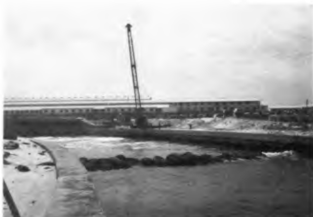
8: TEMPORARY WEIR IN OUTFALL CHANNEL
