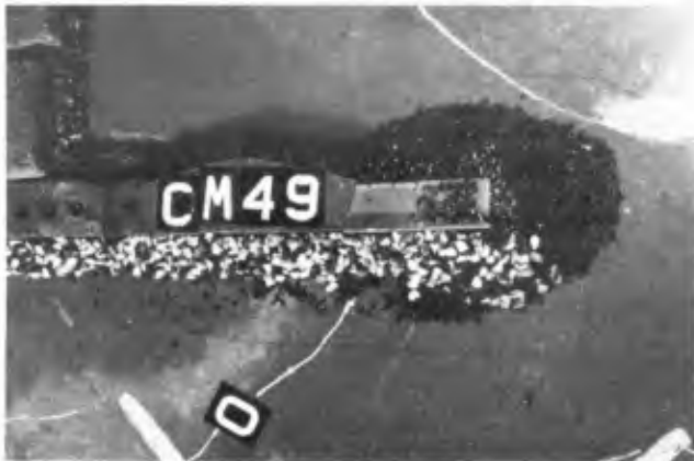
Fig. 3 Damage caused to advancing construction by 3m wave
