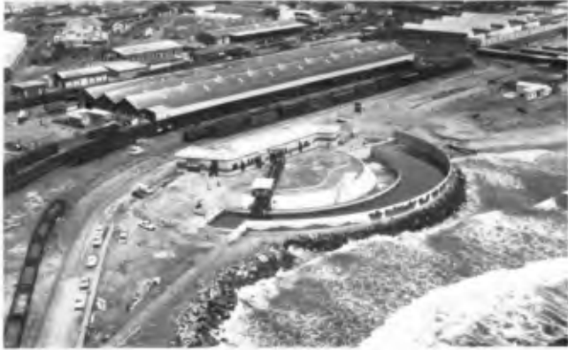
General View of Hopper/Administration Site.
