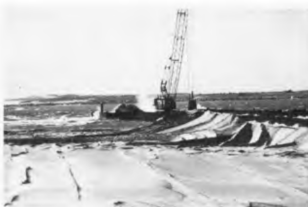
Figure 8 - Pile Driving Activities in Rough Conditions
