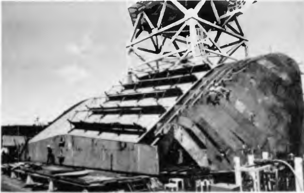
Figure 14 BARGE DURING CONSTRUCTION
