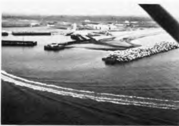
Fig. 7 Build-up in full-size sand trap
