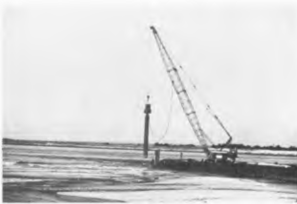
Figure 7 - Pile Driving Equipment
