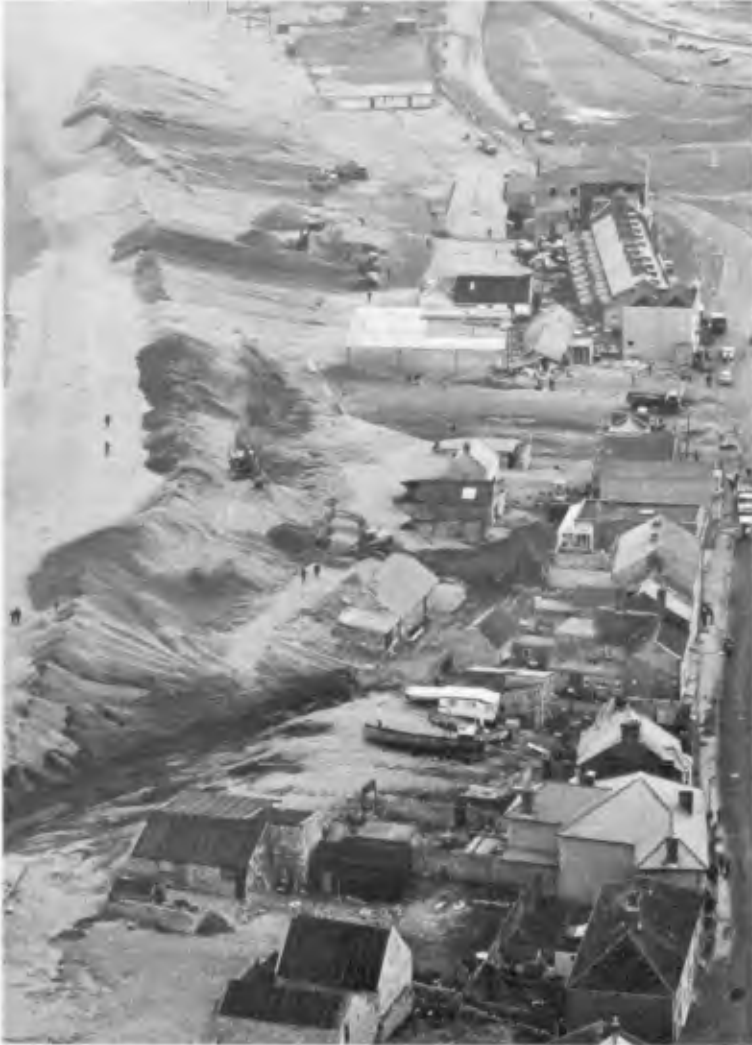
Figure 1 Chesil Beach at Chiswell two days after the flooding. Much material had already been bull-dozed back up to the top of the bank. The sea is to the left.
