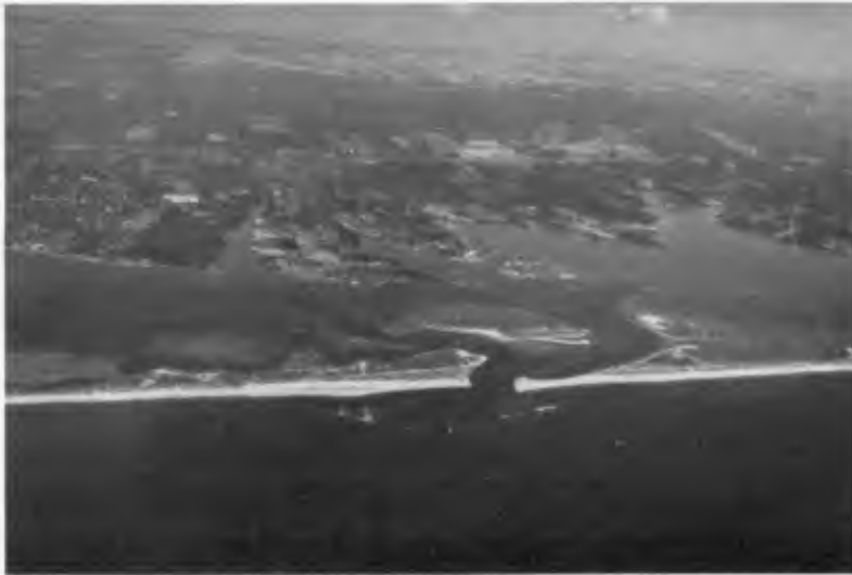
Figure 4 - Moriches Inlet Viewed From the South (September 1973)
