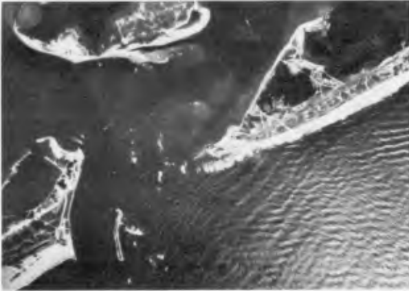
Figure 6 - Initial Construction (10/12/80) (note sheet pile retaining walls)
