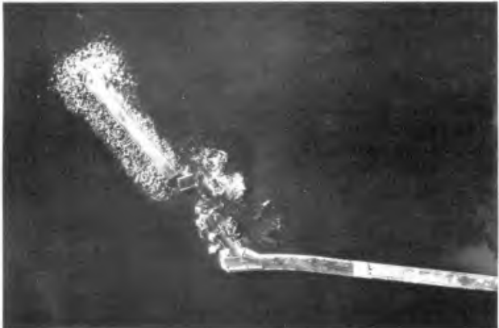
Fig 10. Storm damage to rubble mound breakwater
