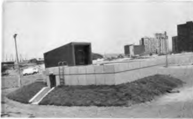
View of Booster Station No. 1
