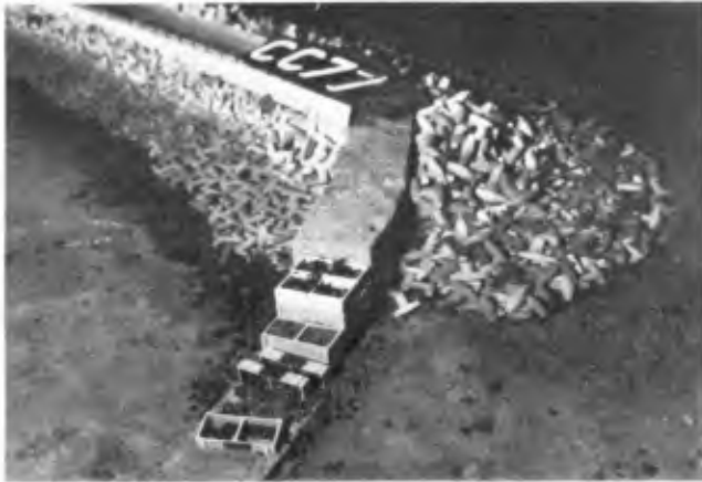
Fig. 8 Model damage to structure in Figure 7 after prototype 4,9m wave impact
