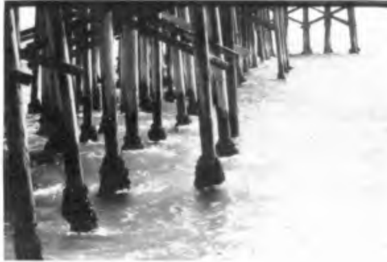
Photograph 1. Pile of Variable Diameter.
