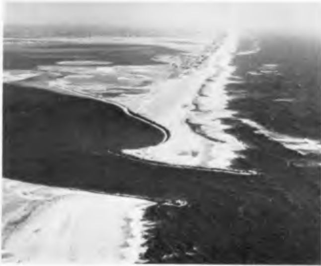
Figure 5 - Pikes Beach Looking East (January 1978)
