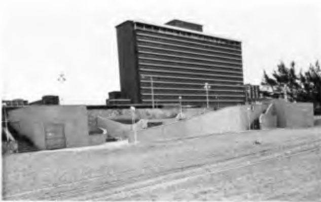
View of Booster Station No. 2
