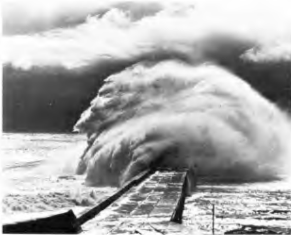
Waves breaking over Gans Bay breakwater
