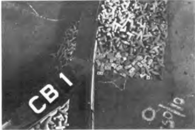
Fig. 11 Advancing face of breakwater protection
