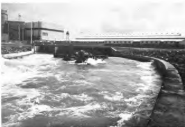
9: COMPLETED WAVE ENERGY DISSIPATOR IN SERVICE
