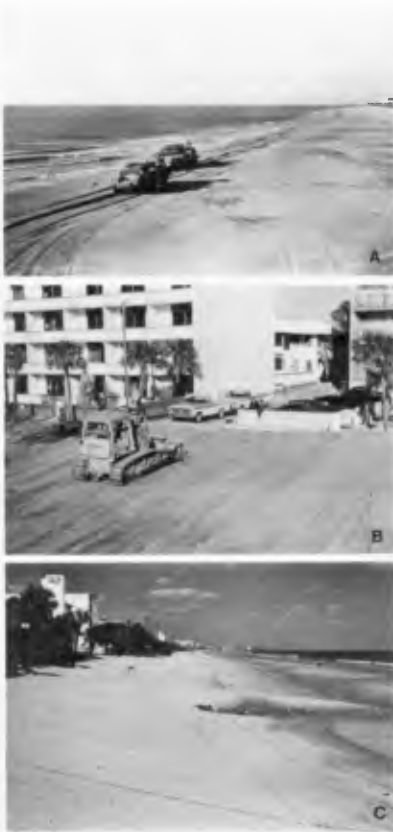
FIGURE 3. (Above) General design for beach scraping and backbeach fill at Myrtle Beach.
