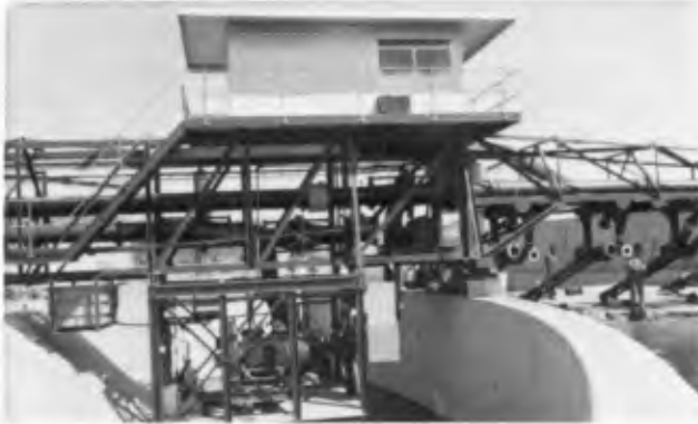
View of Bridge Showing Control Cabin and Underslung Dredge Pump.
