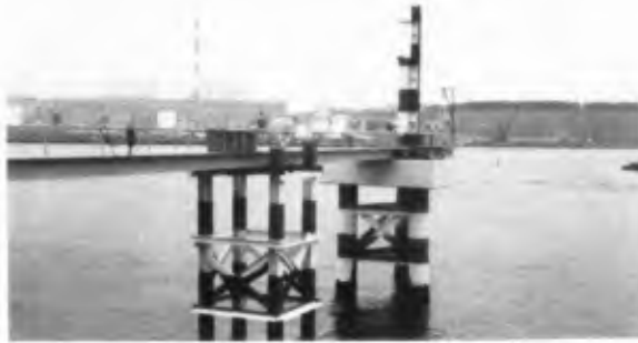
Fig. 2 Monitoring station at the harbor entrance.
