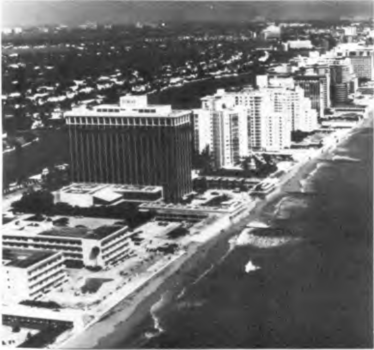
FIGURE 10. Miami Beach, Dade County, Florida, before project construction
