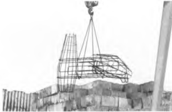
Fig 9. Reinforcing of toe dolos
