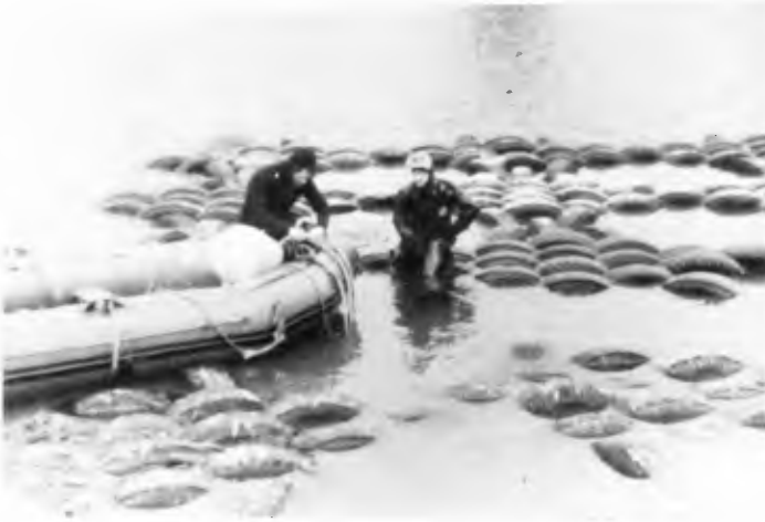
Fig. 7b - Modules with and without buoyance during refurbishing of breakwater
