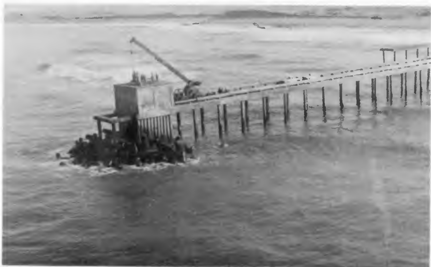
FIG. 4 CLOSE-UP OF DAMAGED DOLOS MOUND
