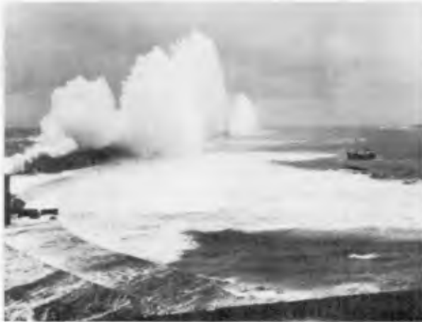
Fig. 15 ALDERNEY BREAKWATER - CHANNEL ISLANDS
