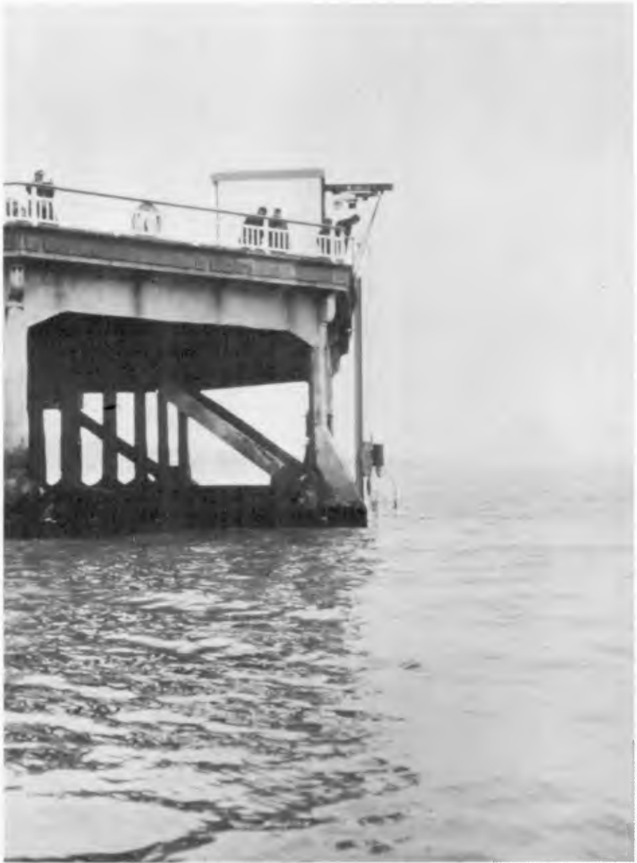
Fig.7 Seaward end of Boscombe Pier
