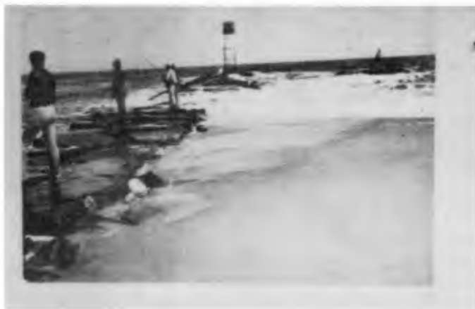
Figure 3 Sand Being Carried Over Indian River Inlet South Jetty by Ocean Waves
