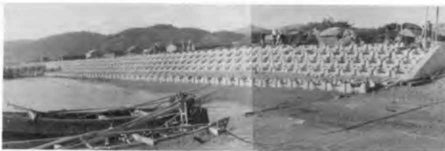
Fig.16 Block faced seadike
