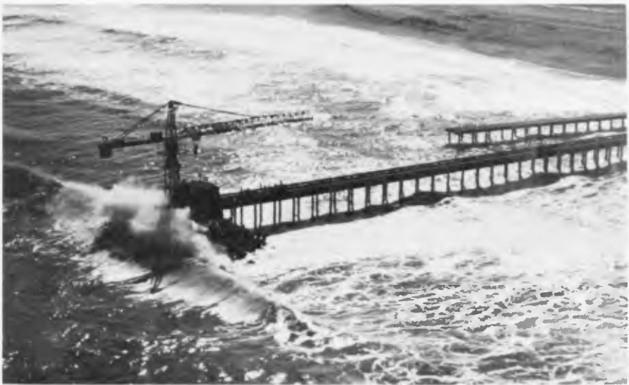
FIG. 12 COMPLETED INSTALLATION, JULY 1978
