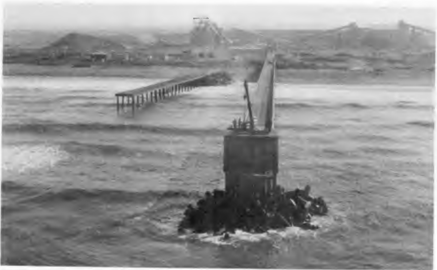
FIG. 2 NEW AND OLD JETTIES WITH DIAMOND RECOVERY PLANT IN THE BACKGROUND
