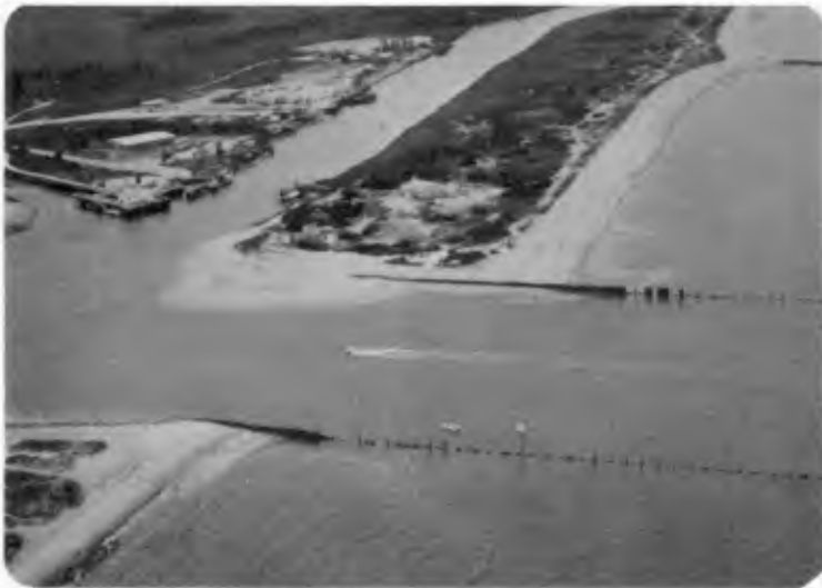
FIGURE 4 Sand easily passing the deteriorated jetties at Roosevelt Inlet and depositing along the western bank.
