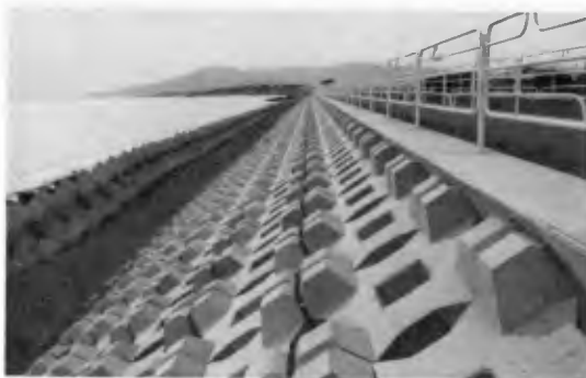
Fig.17 Block faced seawall
