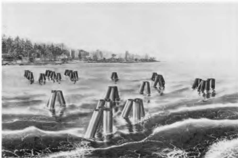
Figure 1 Tripod concept during construction.
