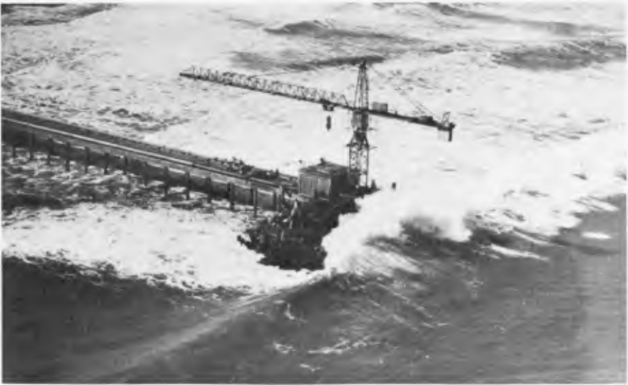
FIG. 11 DREDGE PUMPS IN LEE OF DOLOS MOUND
