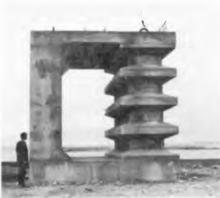
Photo.5-5: Prefabricated Body of Breakwater at Tannawa Marina
