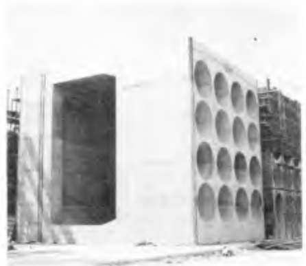
Photo.5-6: Prefabricated Seawall at Kashima Harbour
