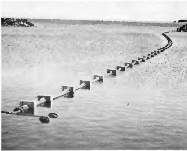
Figure 23. Launching Outfall by String Float Method.
