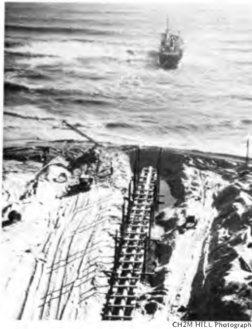
Figure 24. Offshore Tug Preparing for Bottom Pull of Outfall.
