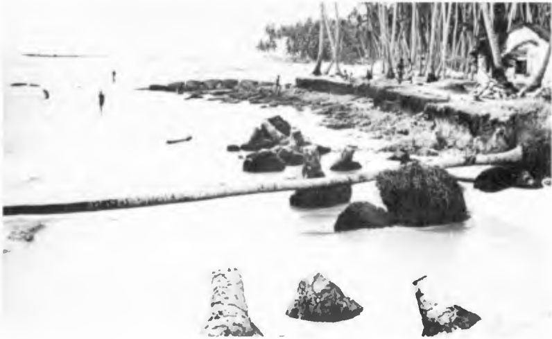
PHOTO 1 SEVERE EROSION ON SOUTHWEST COAST DUE TO COMBINED EFFECTS OF NATURAL CAUSES AND CORAL MINING. NOTE THE REMOVAL OF EXPOSED CORAL.
