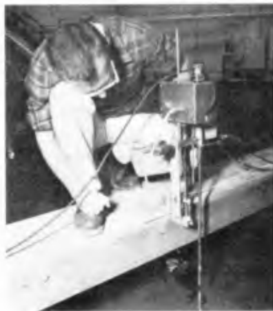
Photo 4. Traversing "Salinity" Probe
