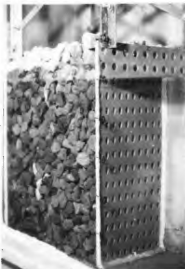
Photo. 2 Rubble Breakwater with Perforated plates
