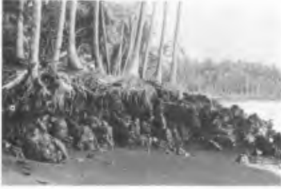
Fig. 7 Underlying lava exposed by beach erosion (1972) (Corps of Engineers)
