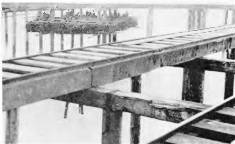
Figure 15. Compressing the mattress.
