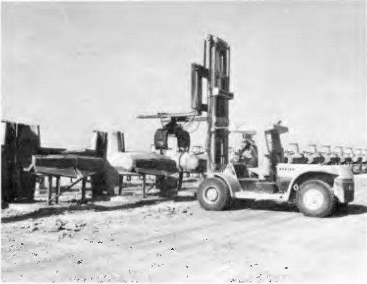
FIGURE 9 Fork lift removing dolos from form
