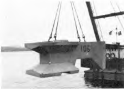
Photo.5-2: A "Warock" hanged by Crane
