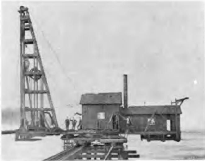
Figure 9. Typical pile driver.
