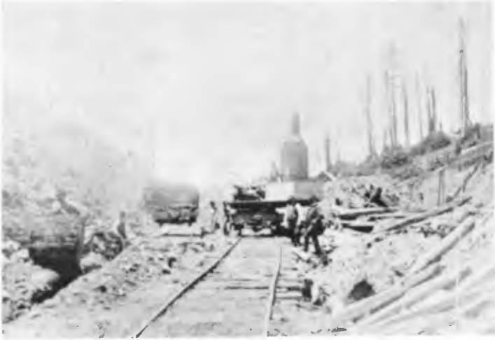
Figure 6. Locomotive crane switching car—Jacoby Creek Quarry.
