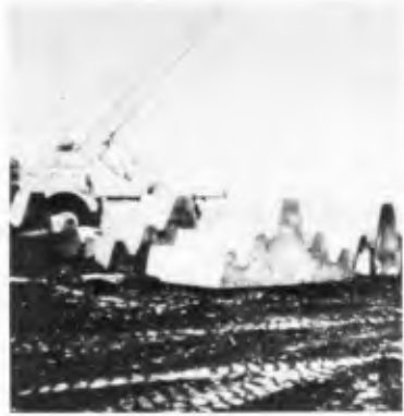
Figure 3. Campbell's precast breakwater units
