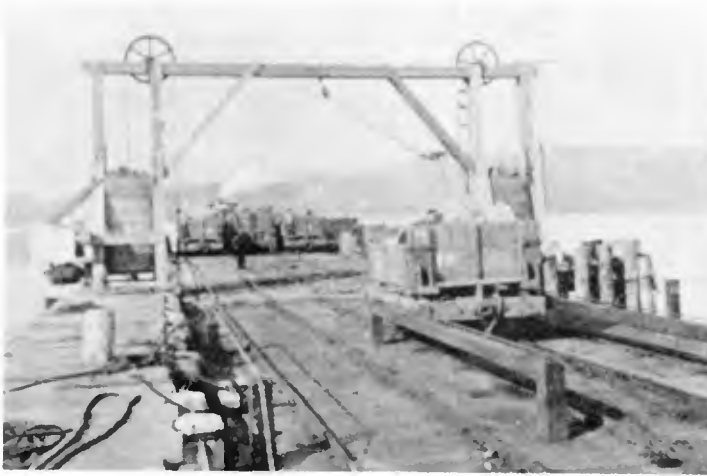
Figure 8. Landing stone at north jetty.
