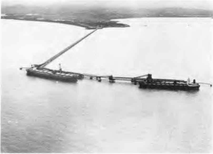
FIG. 1 Hay Point bulk coal loading Berths
