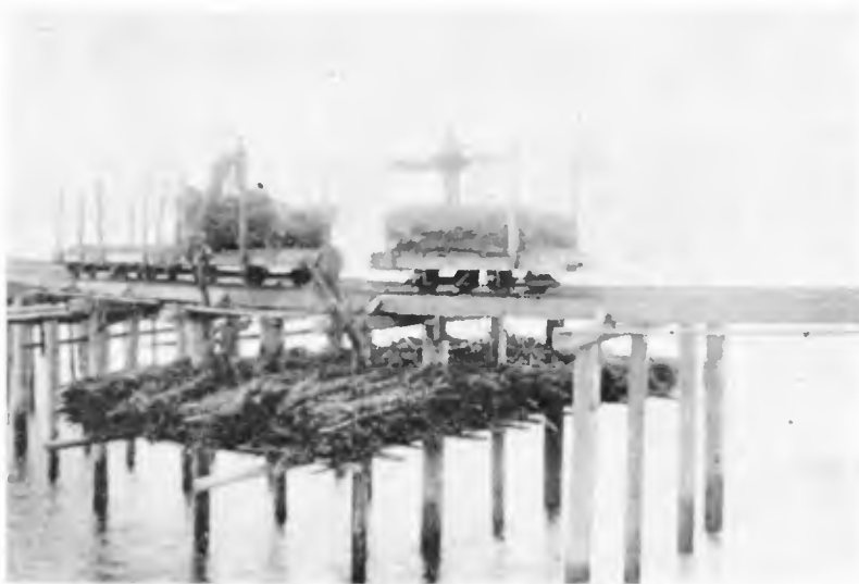
Figure 14. Constructing brush mattresses.
