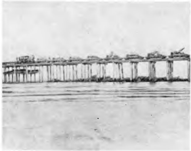
Figure 18. Jetty construction.
