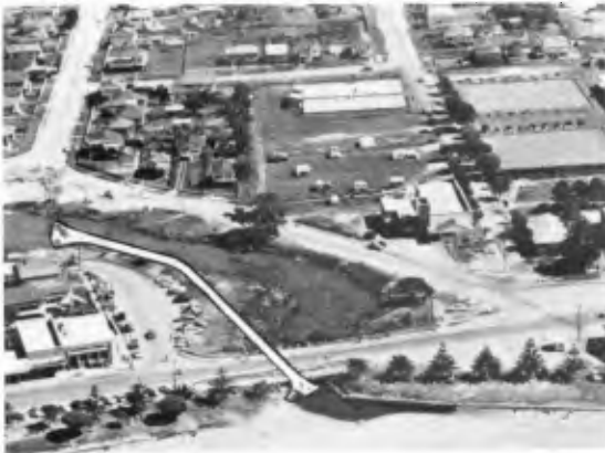
FIG.1. GENERAL VIEW OF REDCLIFFE AND PROPOSED IMPROVEMENT ON THE CREEK
