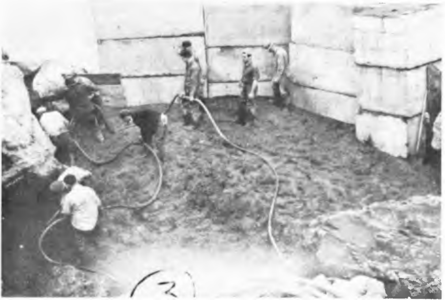
Figure 25. Pouring monolith.
