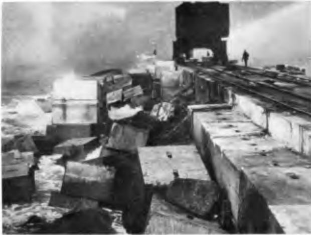
Figure 22. Sea face of south jetty with 20-ton pre-cast concrete blocks (1932).
