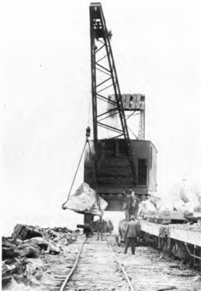
Figure 20. Placing stone from cap.
