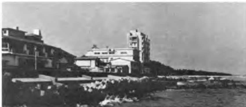
Fig.12 As the wave defence works, armour concrete blocks, named Hexa-leg block, were piled up in front of the seawall. But a number of these blocks have sank under the sea bed ( photo in 1970 ).
