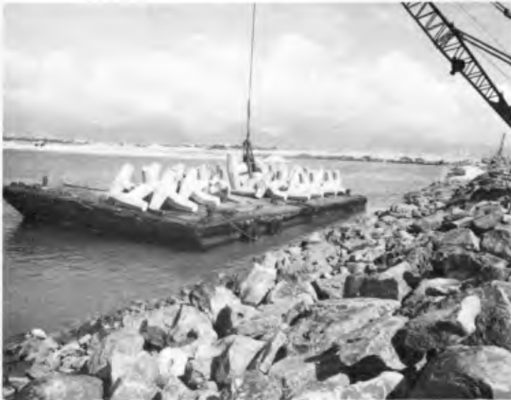
FIGURE 12 Dolosse on barge
