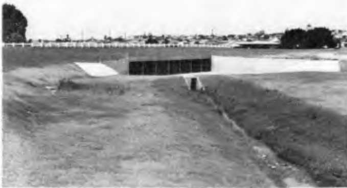
FIG.8. PHOTOGRAPH OF CULVERT ENTRANCE
