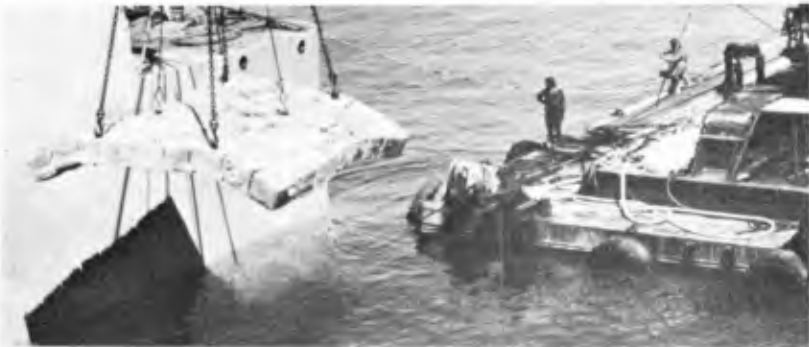
FIG. 14 Laying of scour mat
