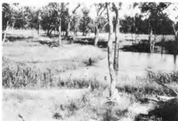
FIG.5. PHOTOGRAPH OF YULEBA WEIR
