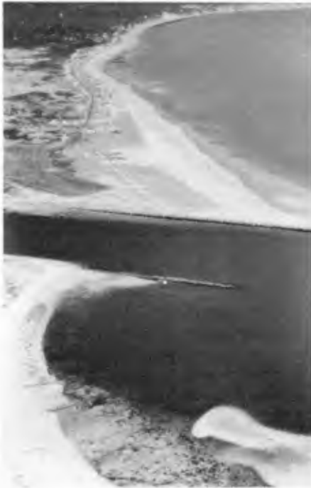
Figure 3. Low tide aerial photograph of the Cape Cod Canal entrance. Note the erosion-deposition pattern resulting from interruption of littoral transport. Sand is moving toward the viewer. Photo by Miles O. Hayes.
