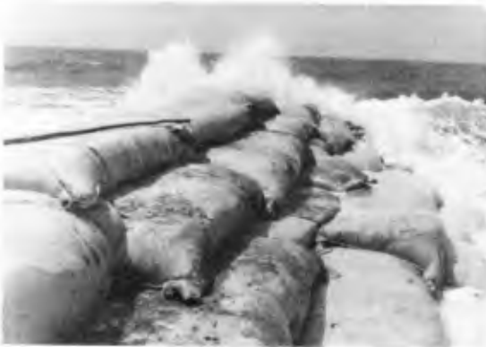
Figure 8. Bolsaroca, large, reinforced, synthetic bags filled with mortar or concrete in sites
