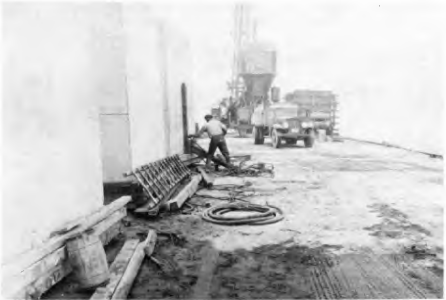
Figure 26. Preparing to launch 100-ton cubes.
