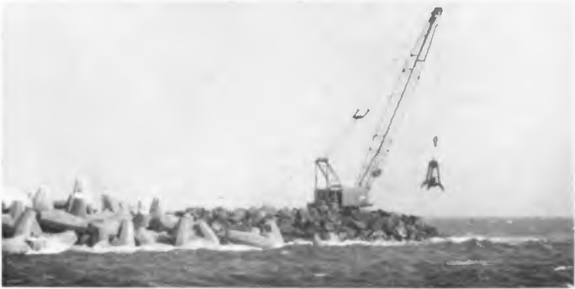
Fig. 6 Breakwater under construction
