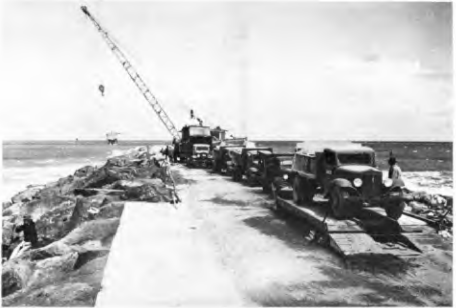
Figure 21. Truck delivery of stone and concrete.
