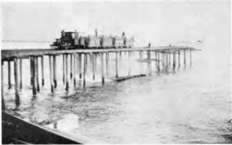
Figure 16. Dropping mattress.
