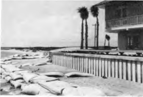
Figure 6. Sand filled bags as a revetment in conjunction with an asbestos bulkhead and dune vegetation at Seabrook Island, South Carolina
