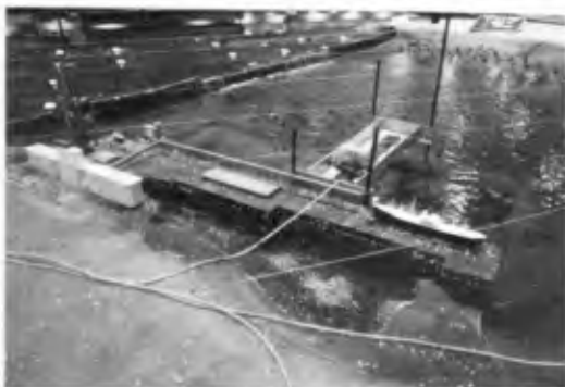
Photo 7. Dam and Weir Upstream of Dock
