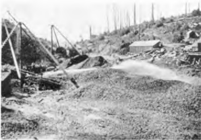
Figure 5. Monitor at Jacoby Creek Quarry
