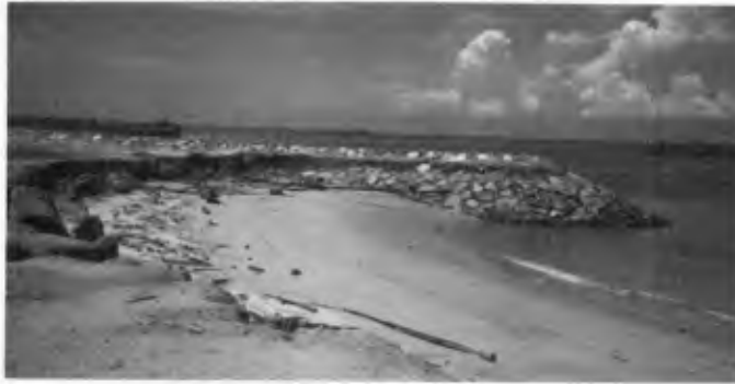
Fig 4 a and b. Rip rap breakwater.
