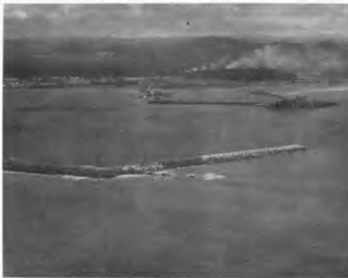
FIGURE 5. Realigned extension of Crescent City Outer Breakwater.
