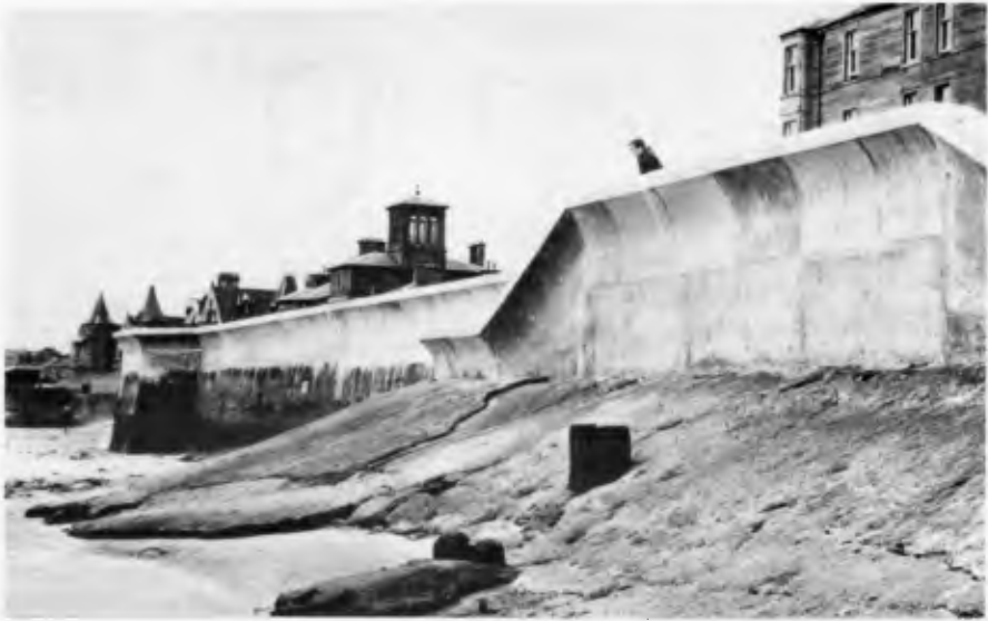
(a) Intermediate Section before replenishment.
