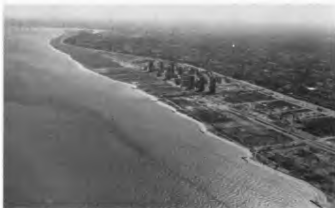
Plate 1. High aerial oblique of Phases I & II Reclamation
