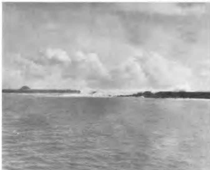
FIGURE 9. Wave overtopping--Crescent City Outer Breakwater.
