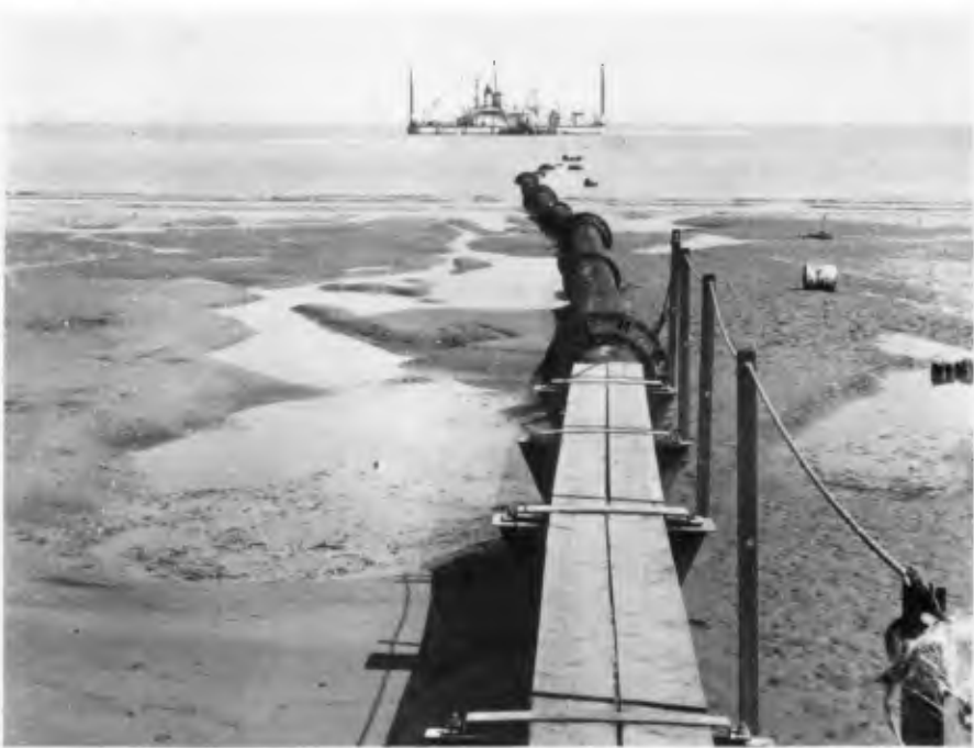
Fig 3. The reclamation dredger and pipeline.
