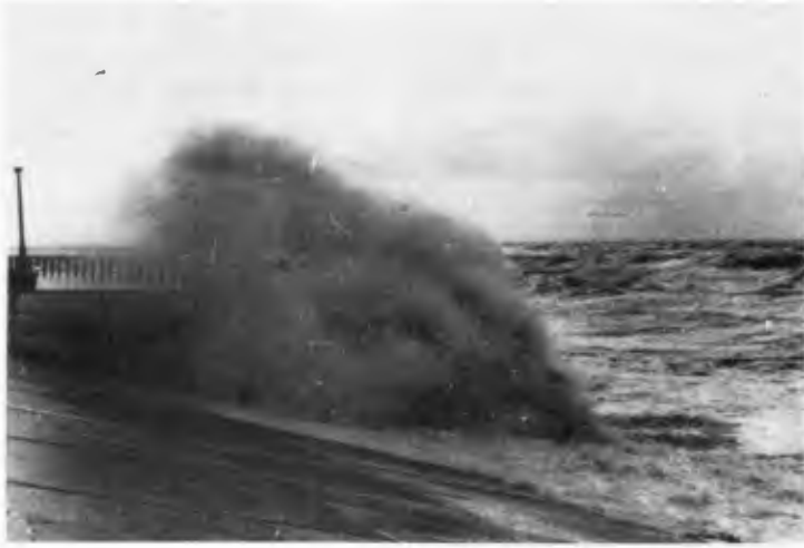
Fig. 6: Wave attack at the seawall of Westerland/Sylt during a storm surge in 1954 (after LAMPRECHT 1955)
