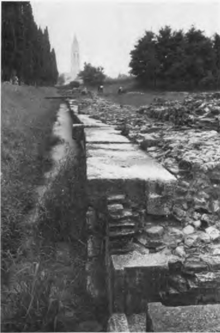
Figure 7. Stone quay in river port of Aquileia, Italy (circa 180 B.C.). Quay had landing stages at two levels (for varying river levels?). Note protruding mooring stones shown in Figure 8.
