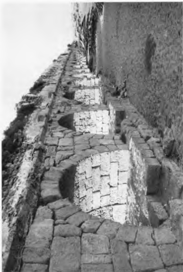
Figure 9. Roman arches supporting the aqueduct leading to Caesarea, constructed about 20 B.C.. Staggered double rows of underwater arches were a favored method of breakwater construction by the Romans.
