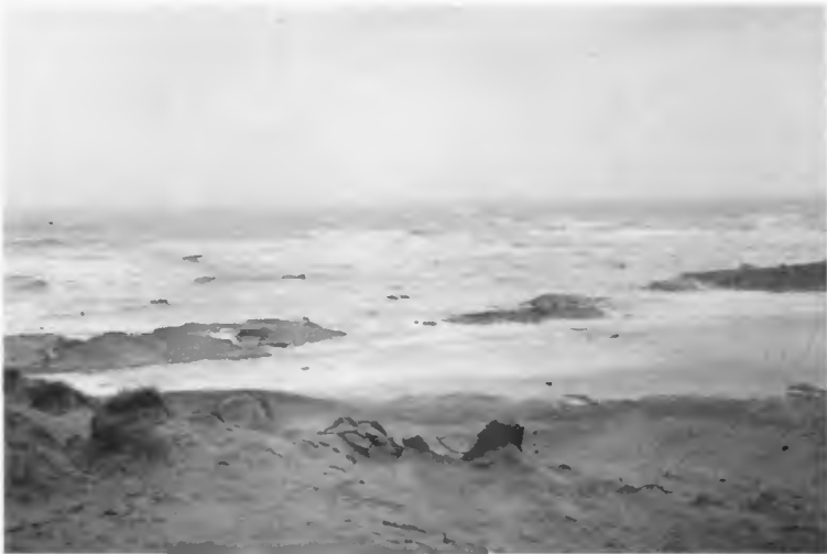
Waves breach deflated remnants of frontal dune protecting large blow-out at Lifeboat Road (Fig.4).
