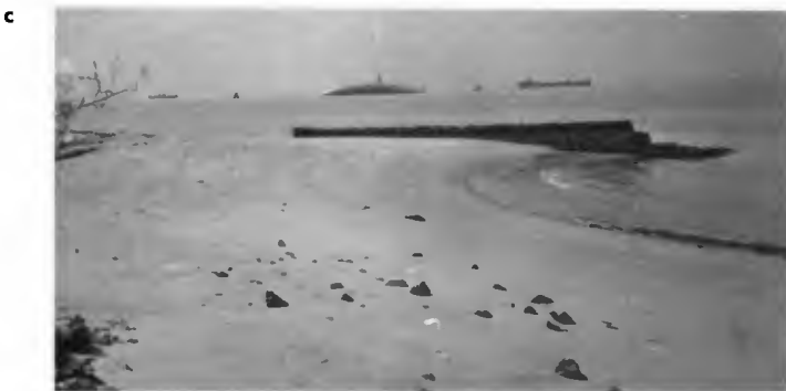
Fig 3 a, b and c. Gabion breakwater
