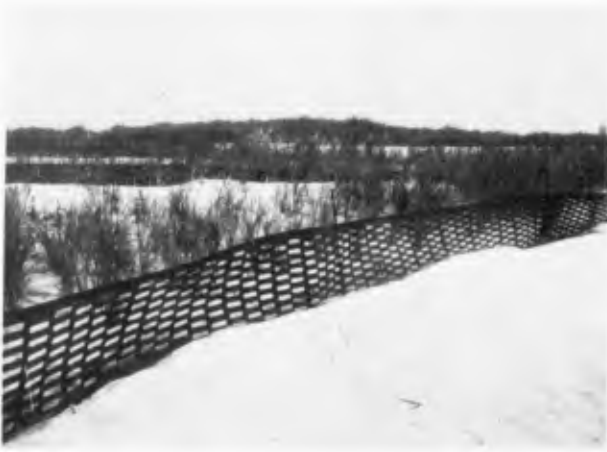
Fig. 6 Sandfence of polyethylene
