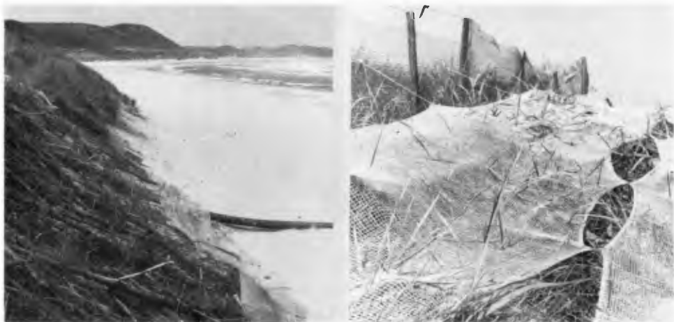
Dune face showing low-cost thatching in July 1973 and the same area in May 1974 with Marram and Sea Lyme grass coming through the branches and hessian cover.
