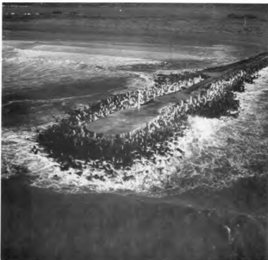
FIGURE 21. Wave dissipation in Dolos armor units--rehabilitated Humboldt Harbor and Bay North Jetty.
