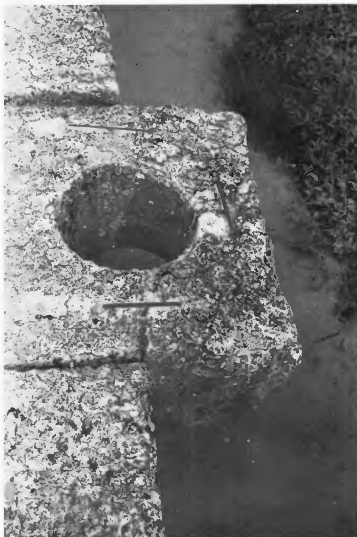
Figure 8. Details of mooring port shown in Figure 7. Port is constructed of three cut stones, morticed together with metal straps.
