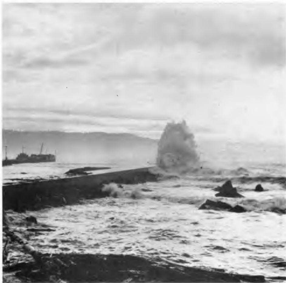
FIGURE 1. Wave attack on Crescent City Outer Breakwater.
