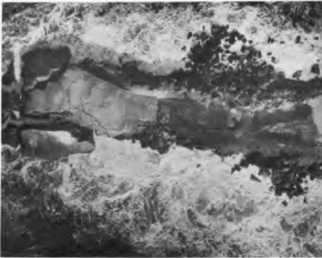
FIGURE 18. Monolithic breakup--Humboldt Harbor and Bay North Jetty.
