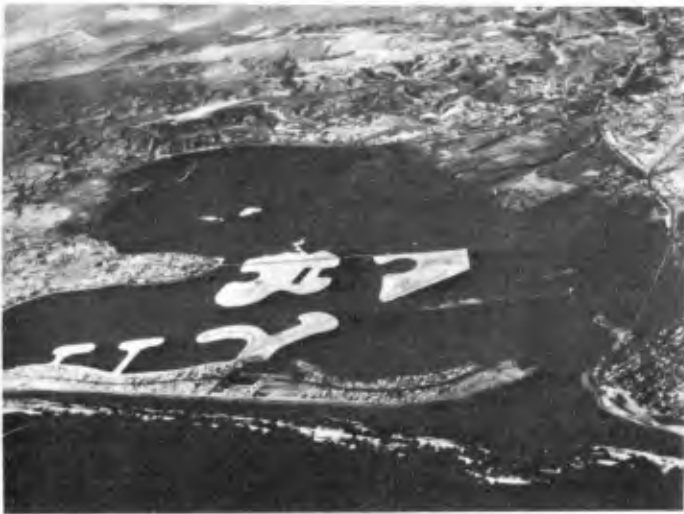
START INTERIOR CONSTRUCTION NOTE CONFIGURATION OF NATURAL INLET FEB. 1948 NO. 2
