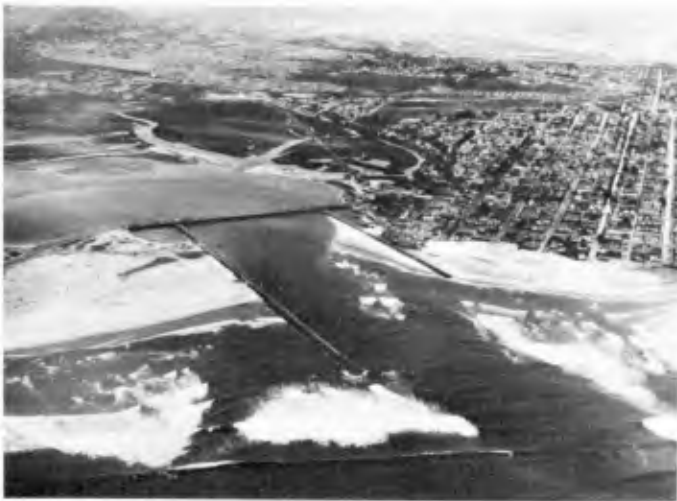
COMPLETION OF FLOOD CONTROL CHANNEL OUTLET MIDDLE AND SOUTH JETTIES FEB. 1949 NO. 4
