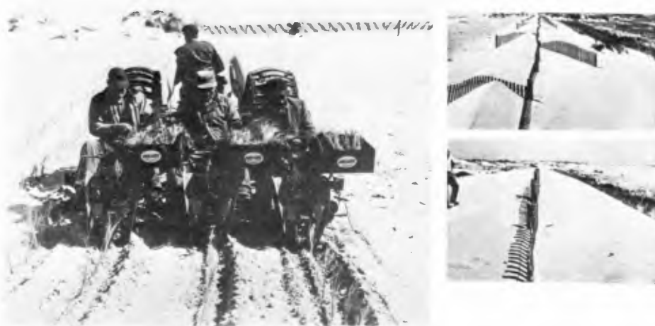
Fig. 24. Dune building by sand fences (NPS, USA)
