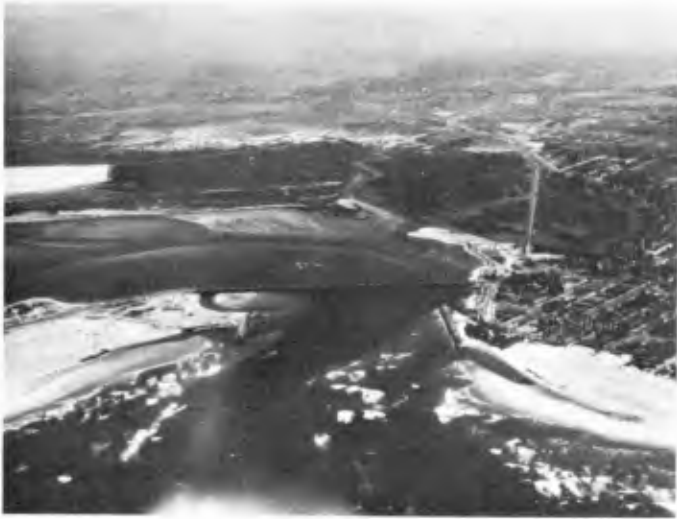
START ENTRANCE CONSTRUCTION MIDDLE AND SOUTH JETTIES JULY, 1948 NO. 3
