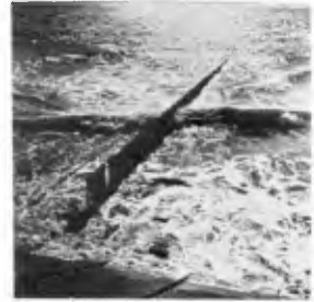
Fig. 12. Dutch groin with piggy back
