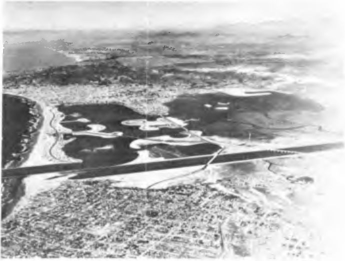
DEVELOPMENT OF WEST MISSION BAY NOTE CLOSURE OF FLOOD CHANNEL JAN. 1953 NO. 7
