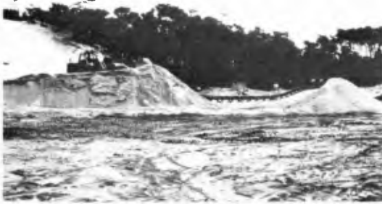
FIGURE 7. Transportation of sand from mining site to plant via conveyor belt.
