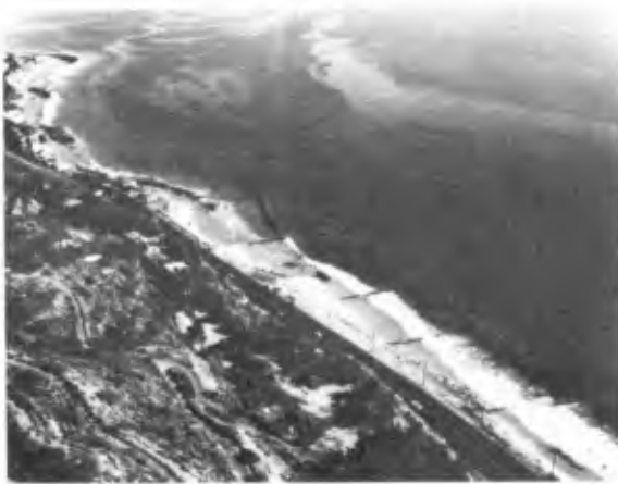
BEFORE BEACH IMPROVEMENT
