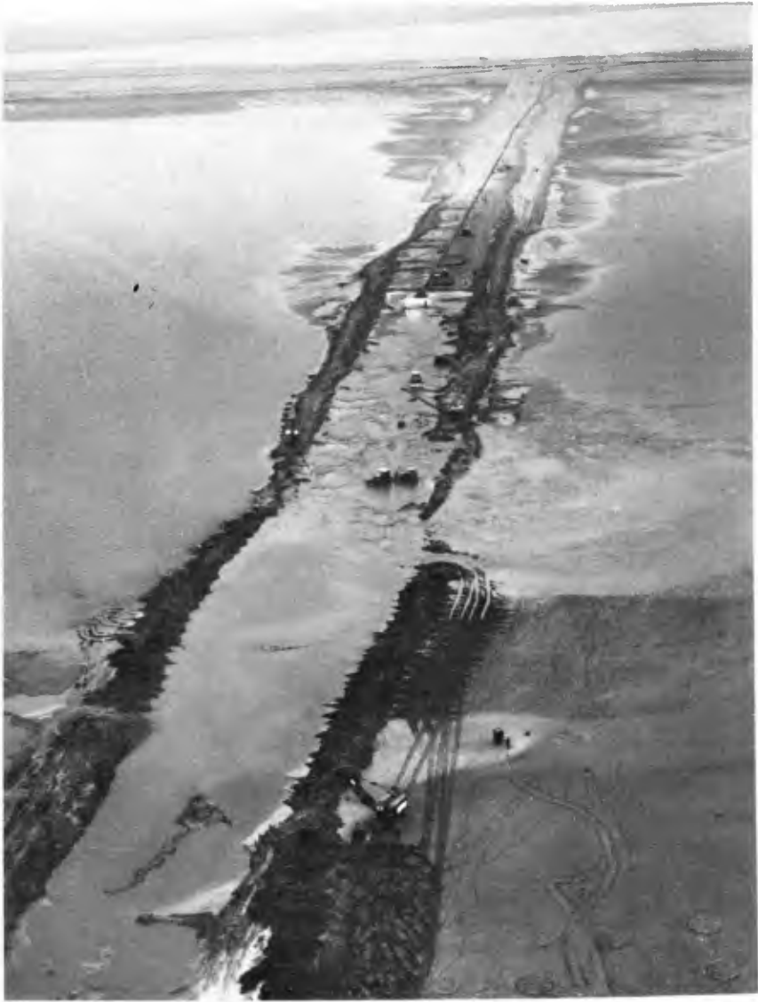
Photo 1. Final gap. Bulldozers and draglines operating on the fill
