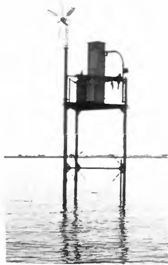
Fig. 10 SILT GAUGE STATION IN THE TIDAL FLAT
