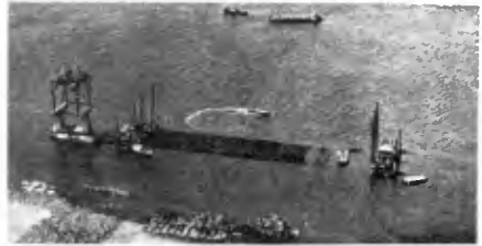
Fig. 10. Placement of zinkstuk of synthetic materials. (Deltawerken No. 58, 1971)
