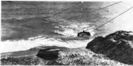
Fig. 53. Artificial nourishment by dragscraper on Jupiter Island, Fla. (Bruun, 1967)
