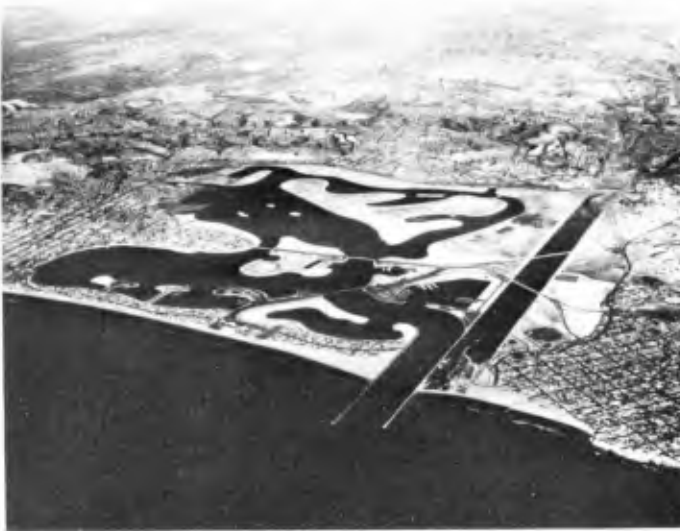
COMPLETION OF MISSION BAY - SAN DIEGO RIVER PROJECT 1963 NO. 9
