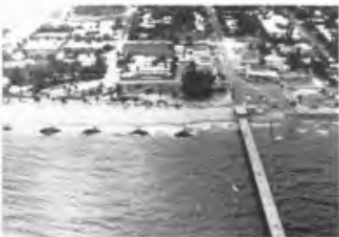
Fig. 47. T-groins at Deerfield Beach, Fla. (Bruun and Manohar, 1963)
