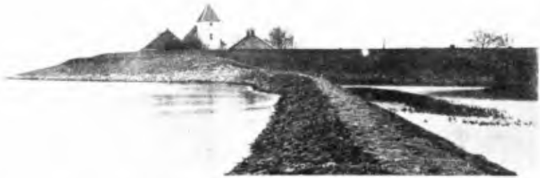
Fig. 1. "Golden Hoop" in the Netherlands. Currentbreaker of later date in front (van Veen, 1962)
