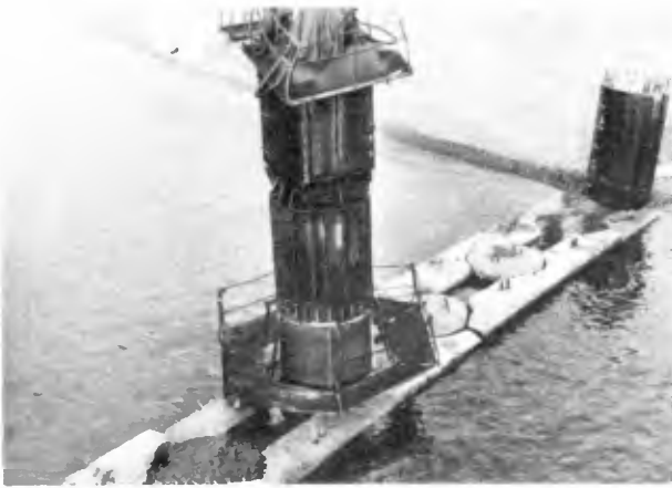
Fig. 3. Groyne made of concrete blocks under construction.
