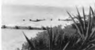
Fig. 41. Adjustable groin at South Palm Beach (Greiser)
