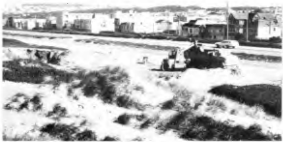
FIGURE 6. Removal of sand using front-end loader and dump truck.
