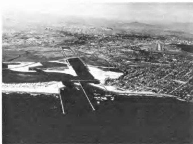
NAVIGATION AND FLOOD CONTROL CHANNEL JETTIES COMPLETION OF NORTH JETTY
