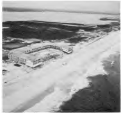
LOOKING NORTHEAST AT ABOUT 3,300 FEET WEST OF GROIN NO. 1
