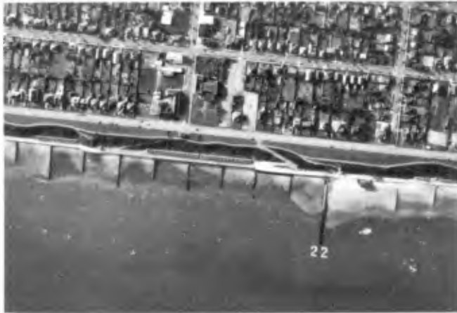
Fig. 5: Part of the frontage with groyne No. 22
