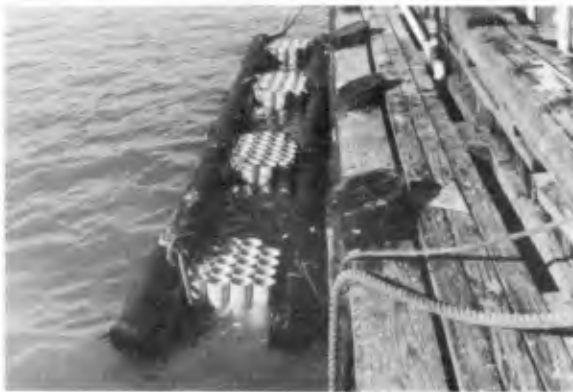
Photo No. 1.-Hi-Dro Cushion Camel Prototype.
