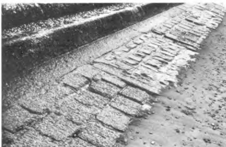
Plate III - Aprons at Dymchurch with granite and concrete blocks as wearing surfaces
