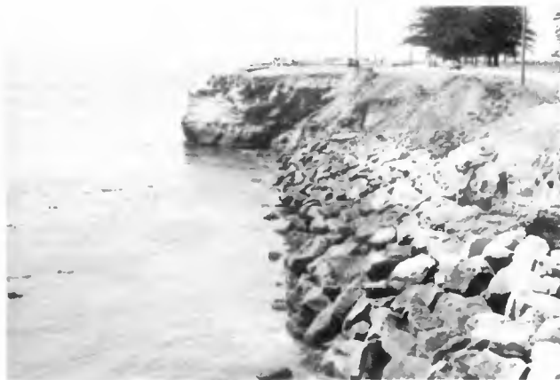
FIGURE 5 - CLIFFS AND PROTECTIVE RIP-RAP SEAWALL AT SANTA CRUZ.
