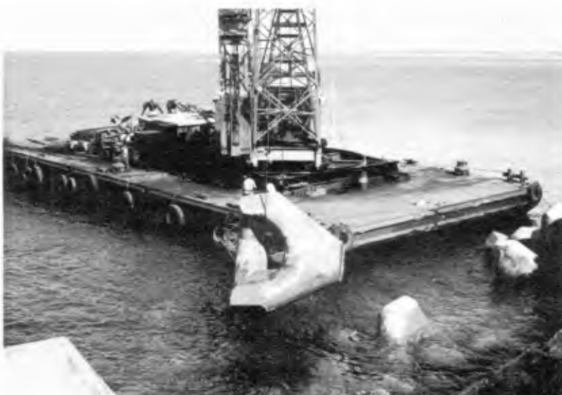
Fig.14 - Floating crane placing Stabitt
