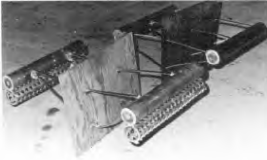
PLATE (1) 'A' FRAME BREAKWATER
