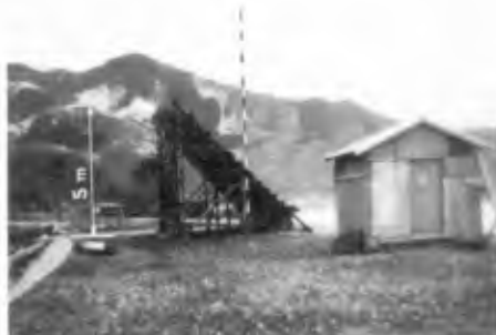
Photo. 1 Facilities of fields observation of wave overtopping at Sakata Coast.
