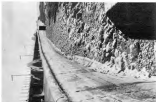
Plate V Abrasion at base of sea wall at Porthcawl
