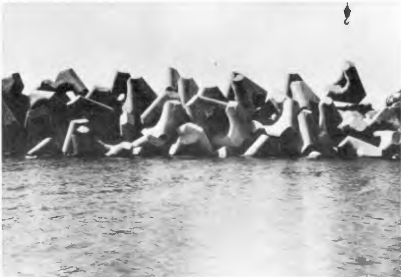
Fig.7 - Stabits placed "brickwall" method
