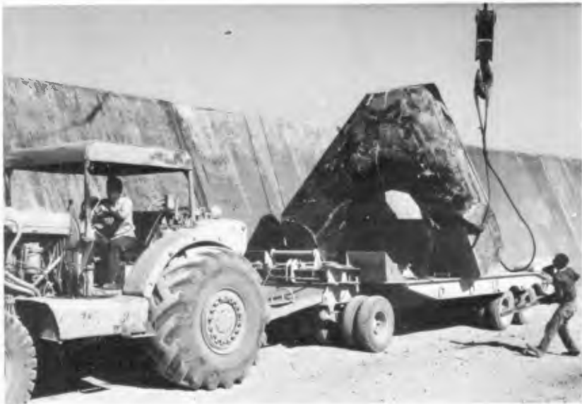
Fig.12 - Low loader transporting Stabit
