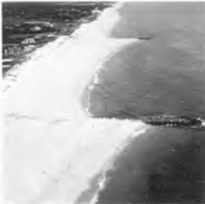
LOOKING EASTWARD FROM WEST GROIN
