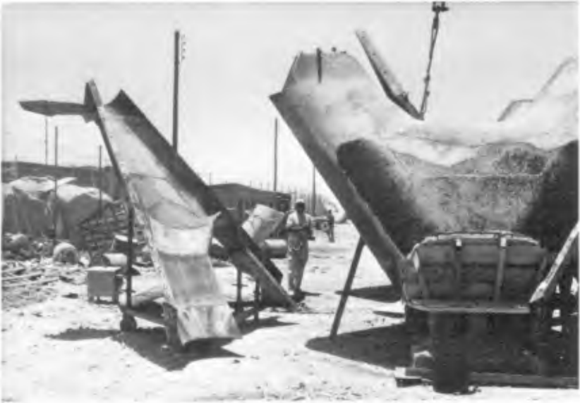
Fig.10 - Stripping Moulds from 29 ton Stab
