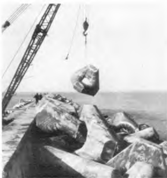
Fig.13 - Lima crane placing Stabitt
