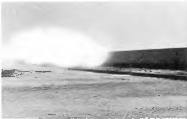
Photo. 2 Conditions of wave overtopping at Oita Coast.
