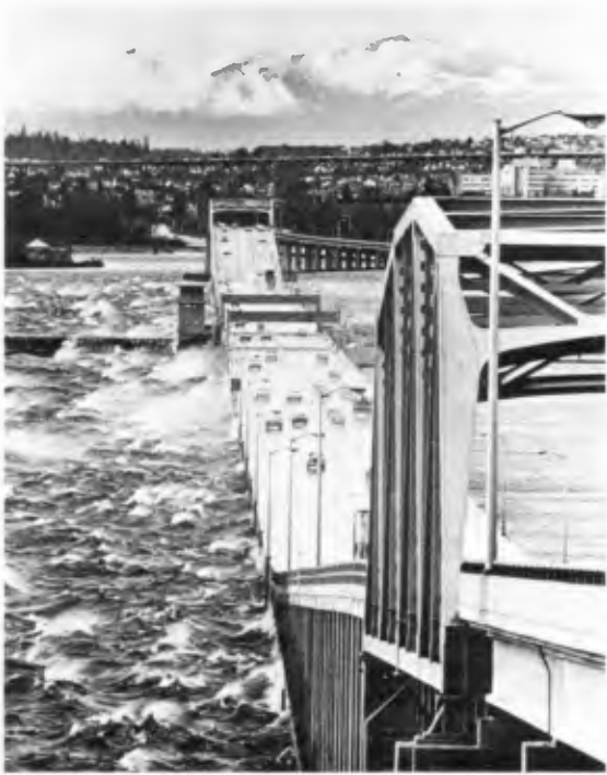
Figure 9. Evergreen Point Bridge U=40\text{mph}
