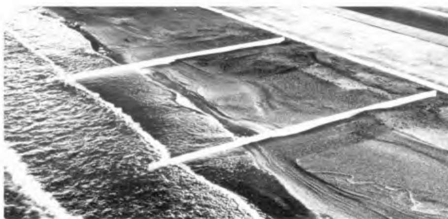
Plate 3. Impermeable Groynes
