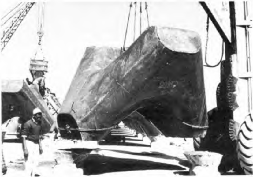
Fig.11 - Stabit being lifted by double sling method
