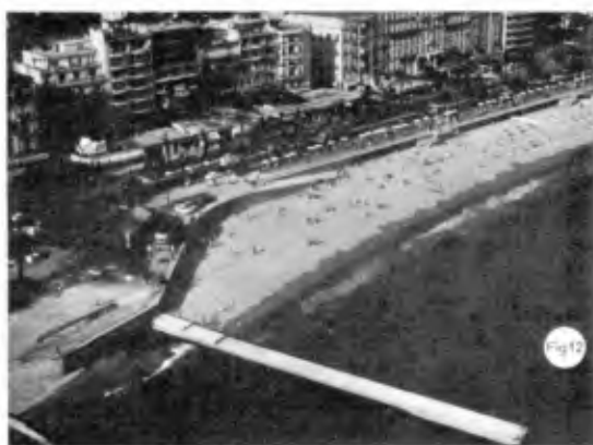
Partitioning jetty (West end)
