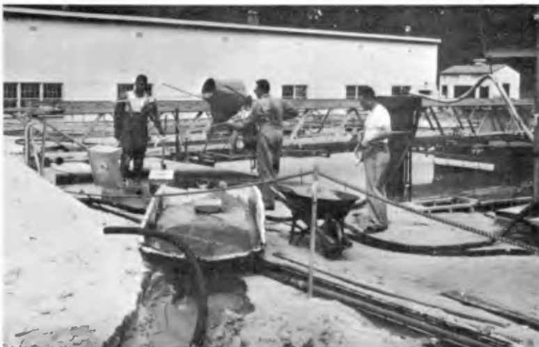
Fig. 4. Tracer Injection Equipment and Technique.
