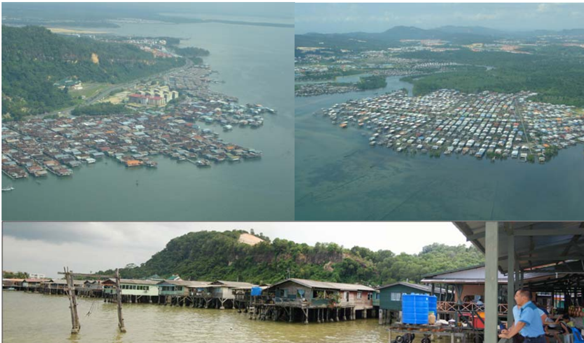
Figure 4. Water villages, consisting of (normally rather flimsy) wooden houses on wooden or concrete stilts are a traditional type of housing commonly found along the coastlines of Sabah, both as small settlements and at the main population centers.
