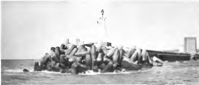
Fig. 3. Breakwater head protected with 19-3/4-ton Dolosse.
