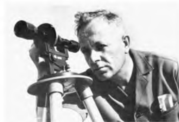
FIGURE 2: WAVE OBSERVATION WITH WAVE CLINOMETER
