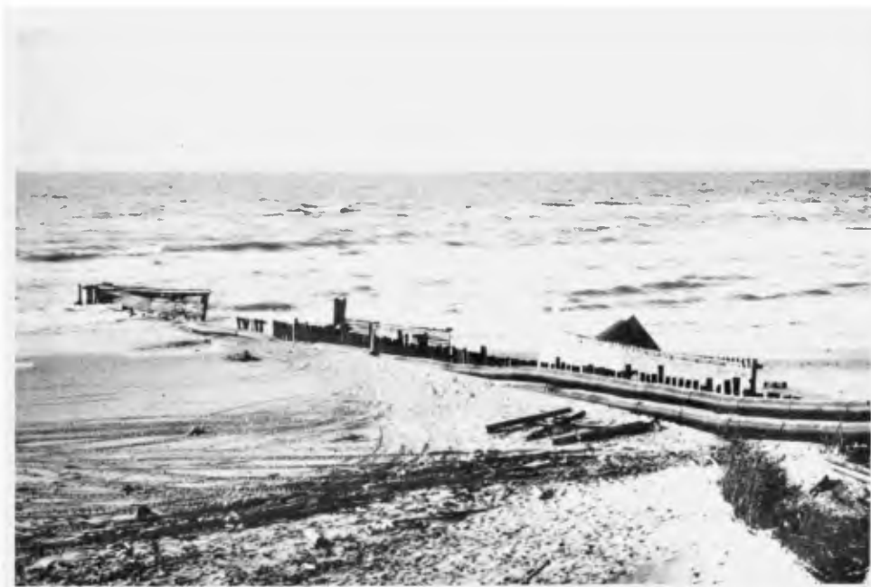
Fig. 4. Sand tube groin (Lønstrup at the Danish North Sea Coast).
