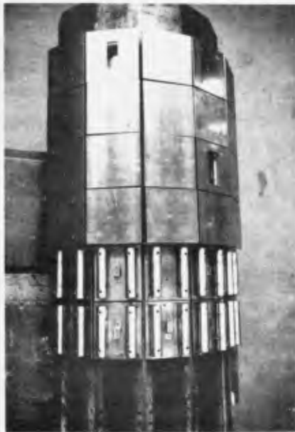
FIG. 4 SHIELD WITH 50 PRESSURE CELLS
