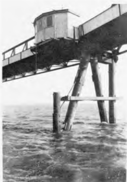
FIG. 5 POINT FOR MEASURING ICE PRESSURE ON A PILE OF A BRIDGE
