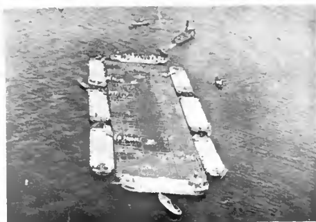
Fig. 9. Towing of willow mattress for bottom protection (van Veen, 1962)
