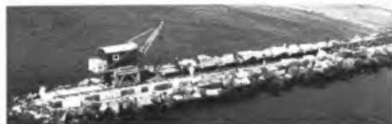
Fig. 43. Groin built of 4-8 ts concrete blocks in the crown and 2-8 ts granite in the slopes. The Lime fiord barriers, Danish North Sea Coast (Hofdahl)
