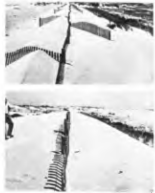
Fig. 24. Dune building by sand fences (NPS, USA)
