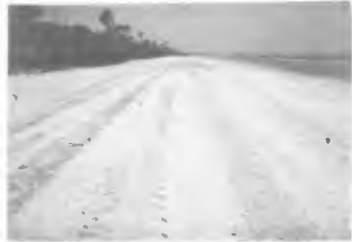
Fig. 49 a and b. Artificial nourishment from land sources, 1,6 mill cu yds on 16,000 ft of shore, Hilton Head Island, S.C.
