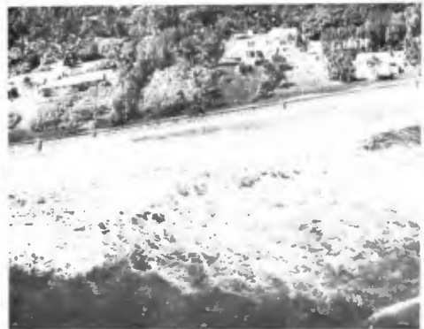
Fig. 37. Interlocking block revetment on Jupiter Island under heavy wave attack (Bruun and Manohar, 1963)
