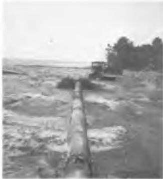
Fig. 49 a and b. Artificial nourishment from land sources, 1,6 mill cu yds on 16,000 ft of shore, Hilton Head Island, S.C.
