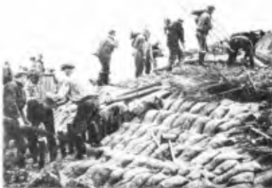
Fig. 4. Polder boys repairing dike with willow, Netherlands (van Veen, 1962)
