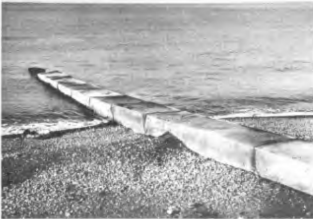
Fig. 4. Groin made of concrete blocks is fully completed.
