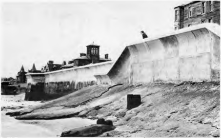
(a) Intermediate Section before replenishment.
