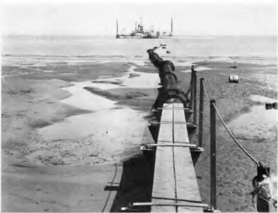
Fig 3. The reclamation dredger and pipeline.
