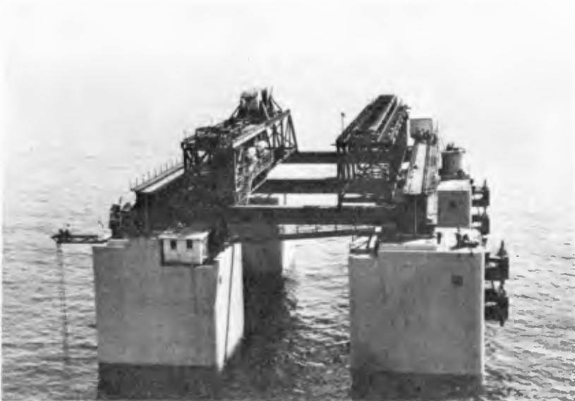
FIG. 4 Main Berth Caisson grounded at Hay Point
