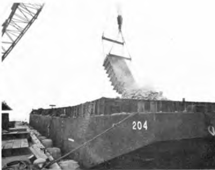
FIGURE 6 Kaunakakai, Molokai Wharf - Crane Loading Barge.
