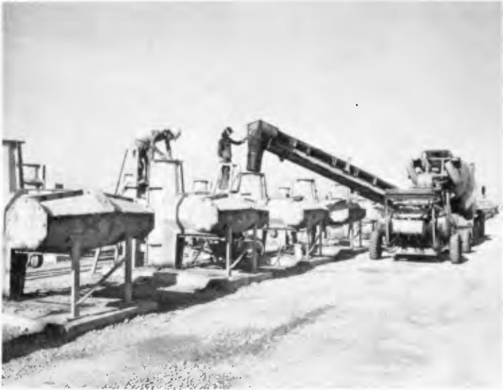
FIGURE 7 Casting Concrete Dolos
