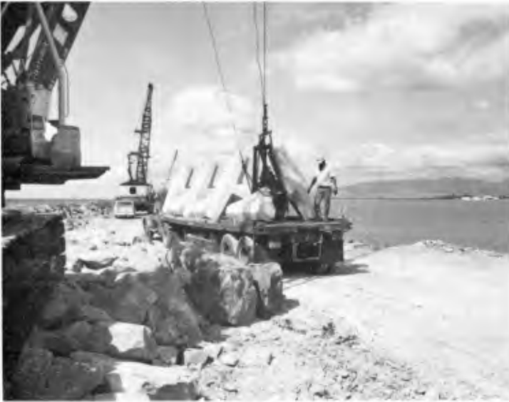
FIGURE 11 Dolosse on flat bed truck
