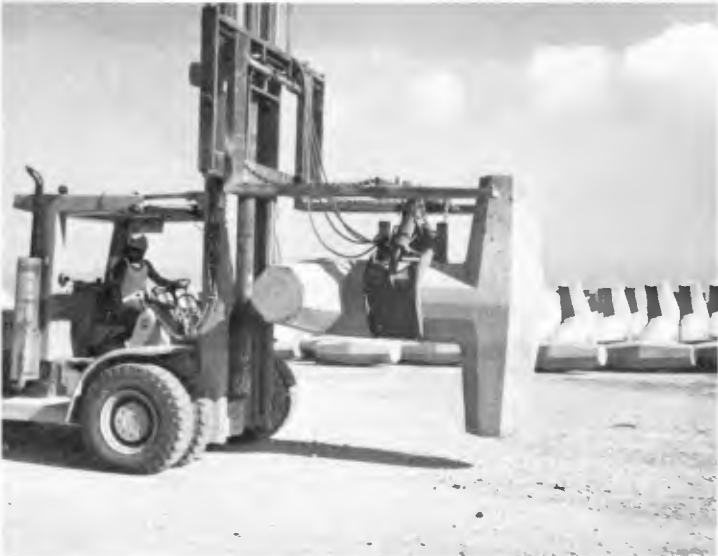
FIGURE 10 Fork lift placing dolos in storage yard
