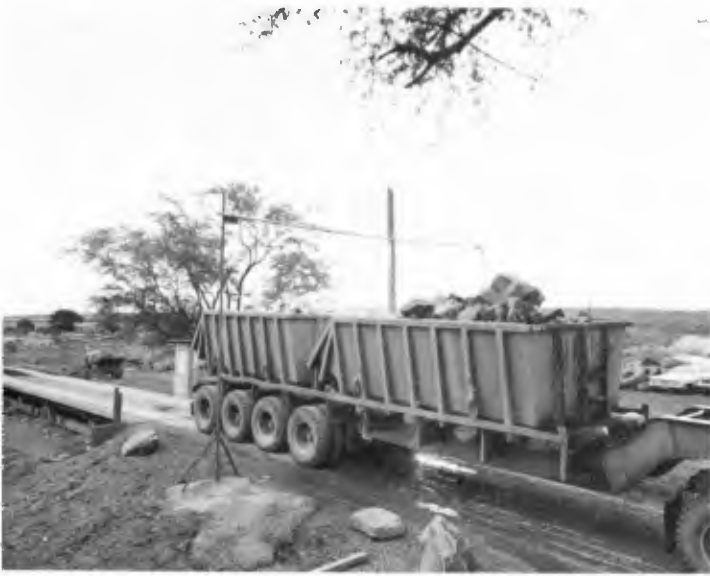
FIGURE 5 Molokai Quarry - Stone Hauling Truck.
