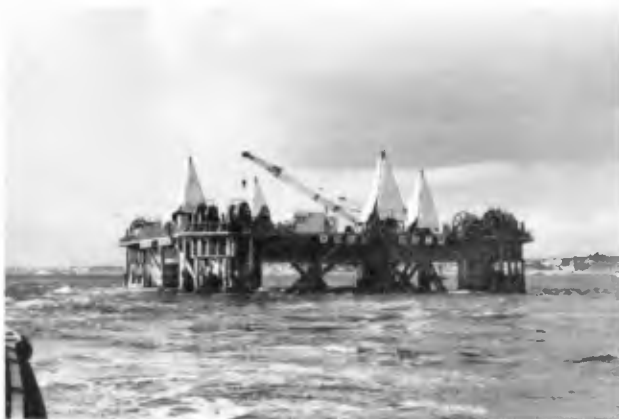
Fig.21. Picture of the floating drilling platform
