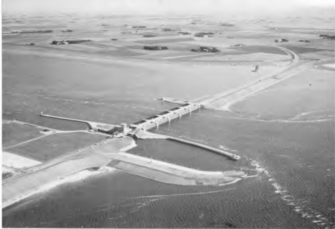
Eider Barrage and Lock
