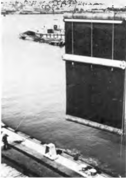
Figure 11 Rigging a curtain section for proper buoyancy
