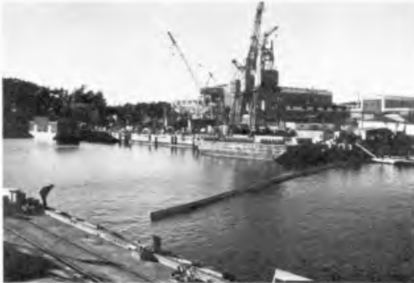
Figure 15 The curtain in the closed and anchored configuration as seen looking into the Pier 20-21 berth
