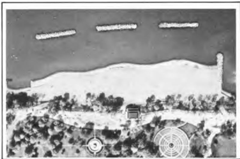
PHOTO 1: IMMEDIATELY AFTER CONSTRUCTION, OCTOBER 1977
