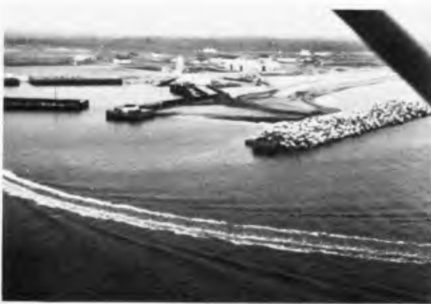
Fig. 7 Build-up in full-size sand trap
