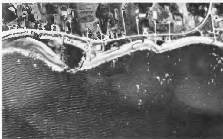
Fig. 2 Harbour before sand trap construction
