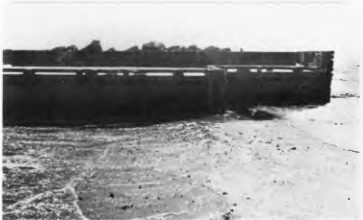
Fig. 3 Sand deposition in harbour entrance
