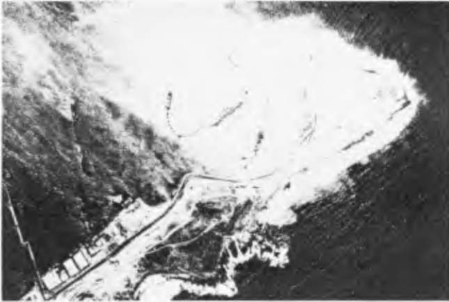
111. 11. Aerial photograph of Hoedjies Point at the beginning of the second building stage.
