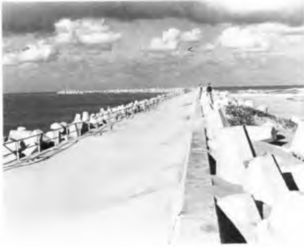
Richards Bay South breakwater
