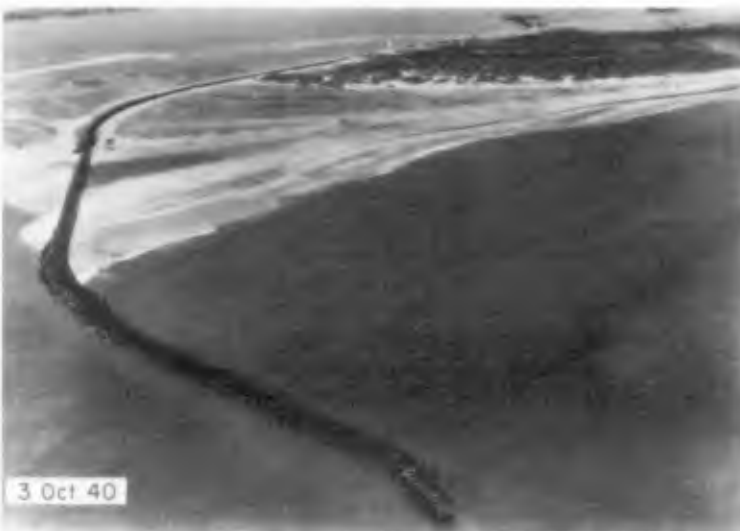
New York Daily News Copyright, with Permission Figure 6. SEGMENT 3 UNDER CONSTRUCTION ON 3 OCTOBER 1940.
