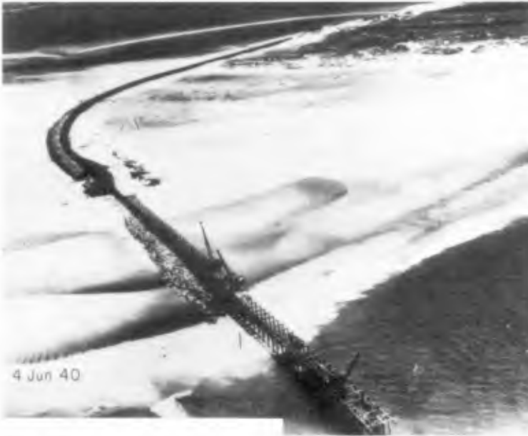
Figure 5. SEGMENT 1 OF JETTY COMPLETE AND TRESTLE CONSTRUCTED FOR SEGMENT 2 ON 4 JUNE 1940.
