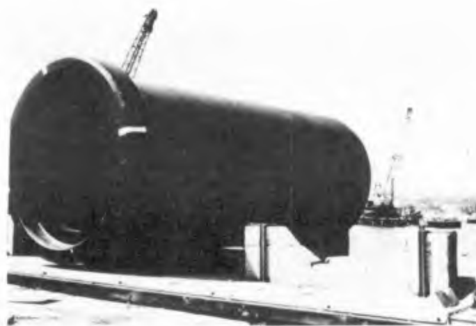
COAL-TAR EPOXY FINISH ON PIPE
