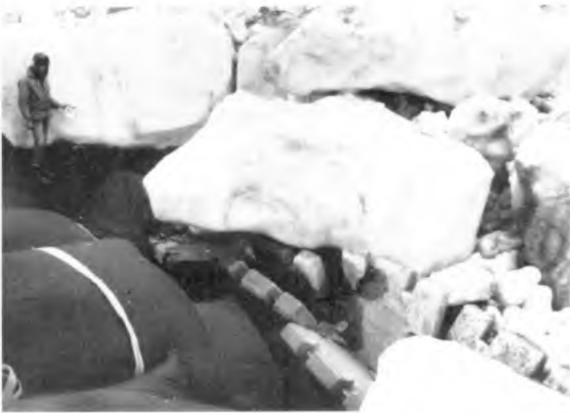
PHOTO 5: BLOCK DISPLACEMENT BY LARGE ICE IMPACT, AUGUST 1988
