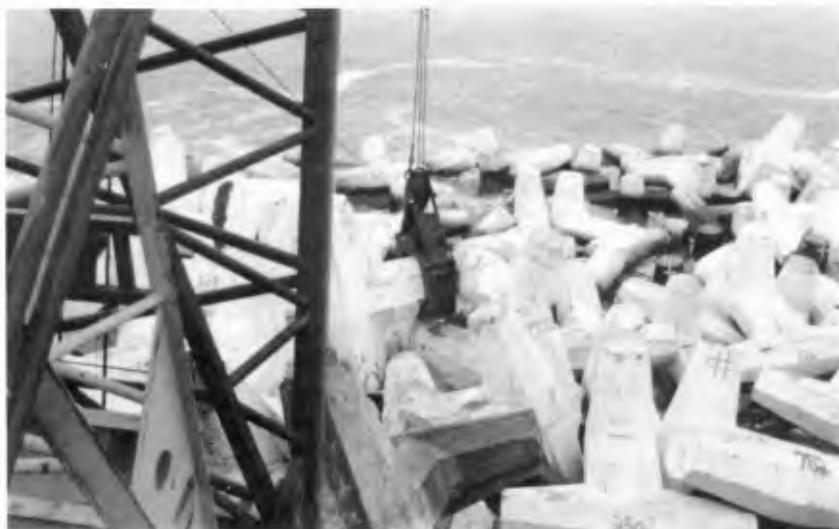
Figure 1: 38-tonne Dolosse at Crescent City, CA
