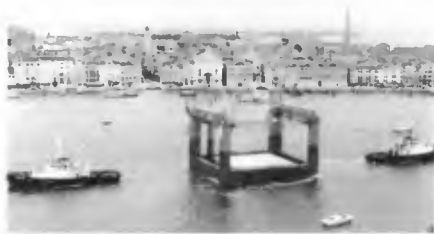
Test Section of Venice Barrier being Transported to Lido Inlet
