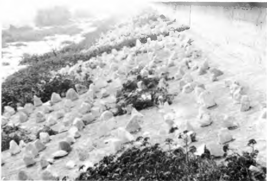
Photo 1-2 Views of the existing murazzi at Pellestrina (in some areas with macro-roughness elements)
