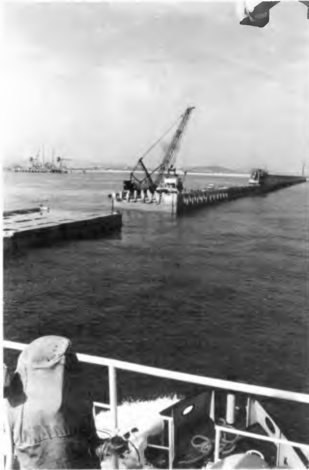
Perforated Caisson Breakwater at Porto Torres, Sardinia
