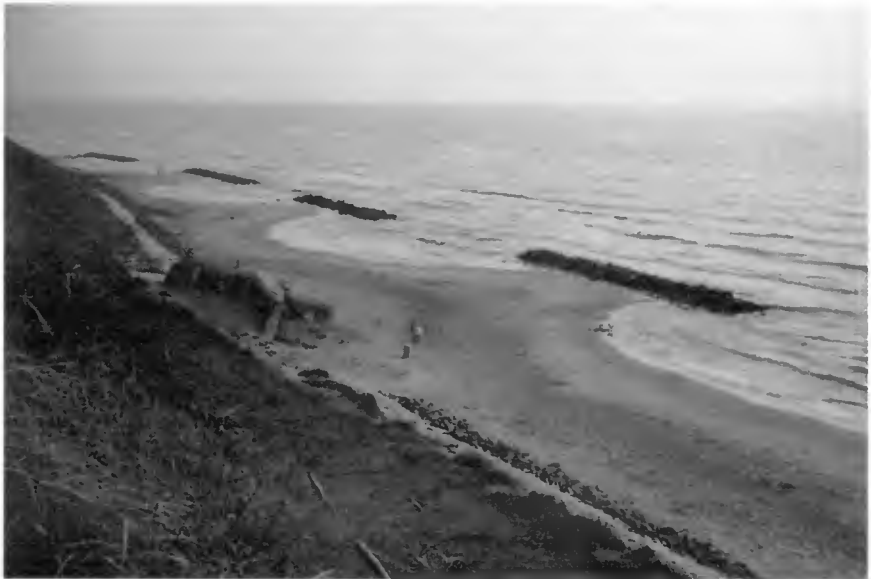
Coast Protection at Lønstrup, Danish North Sea Coast
