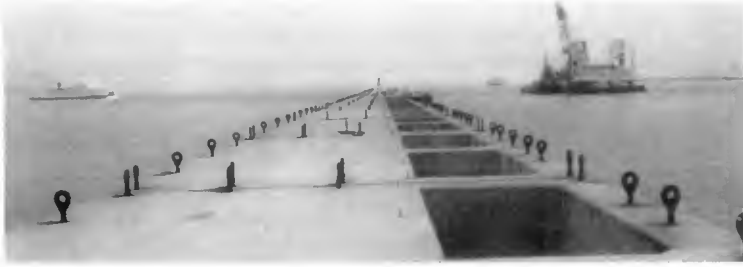
Photo.1 View of slit caisson under construction
