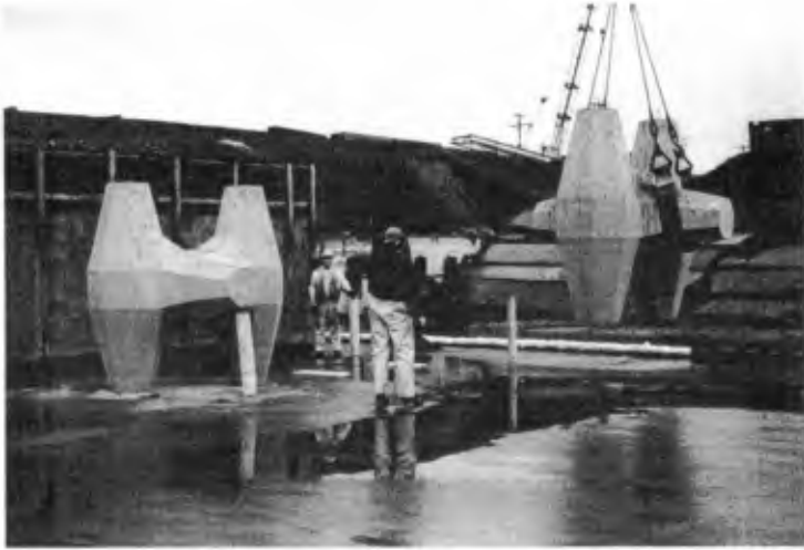
Figure 1. The first 9.2-tonne prototype CORE-LOC™ units
