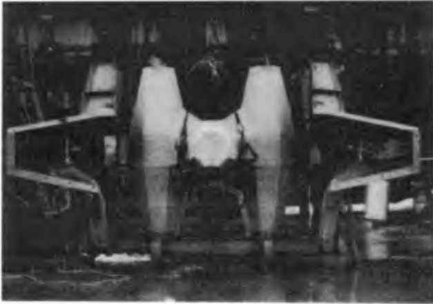
Figure 5. Four-piece "clamshell" mold
