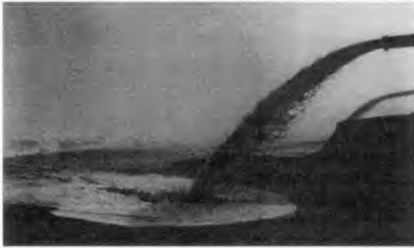
Figure 2: Dredger tailings discharge
