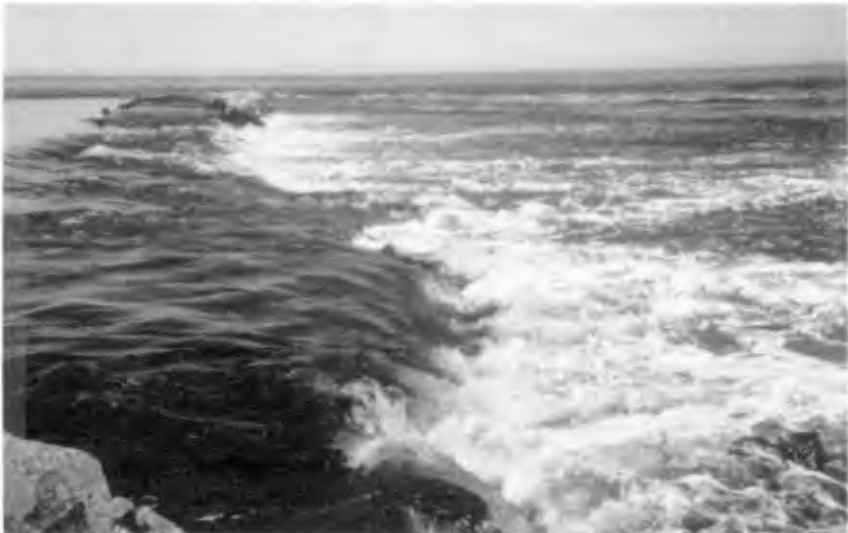
Figure 8. During spring tide after the completion of the construction "road". Note the head difference of about 1 m.
