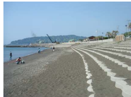
Fig. 2 Sand deposition on steps of gently-sloping revetment on Katsuyama coast.
