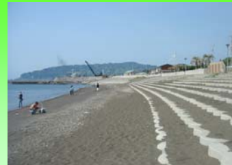
Fig.1 Sand deposition on steps of gently-sloping revetment on Katsura coast.
