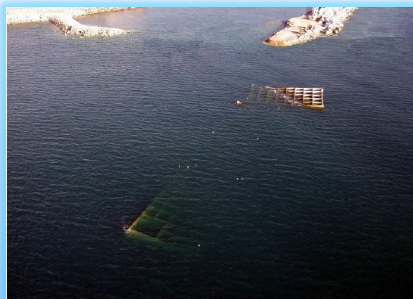
Figure 1. Failed caissons.
