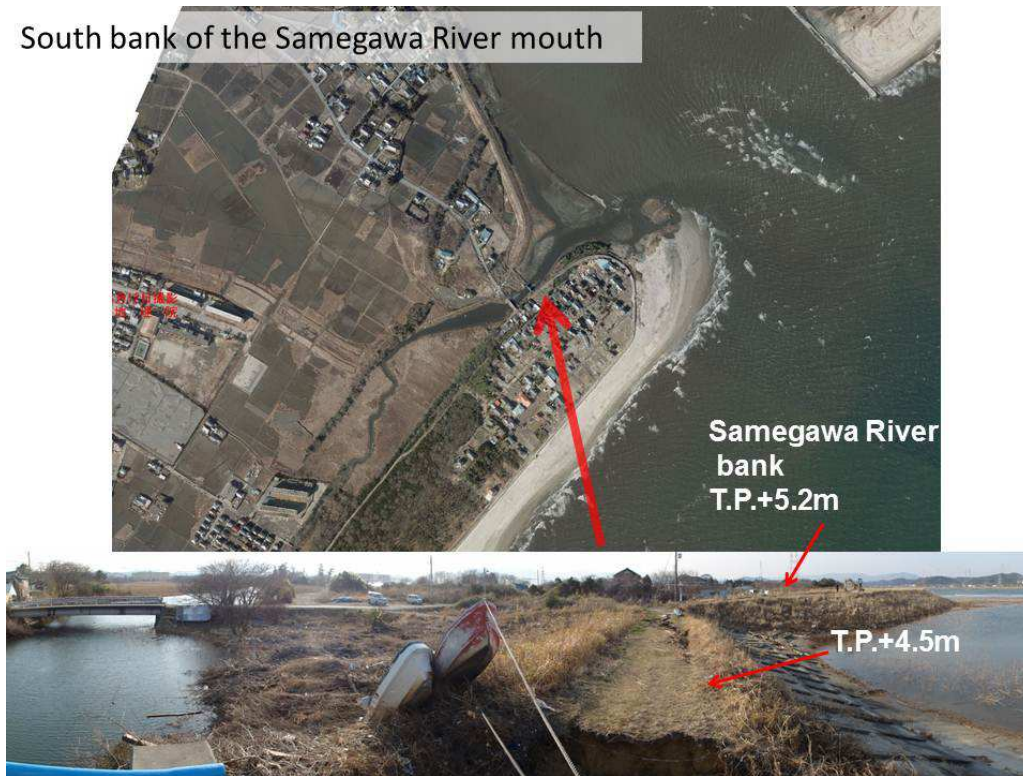
Figure 12. Inundation from broken river bank connected to intact seawall. (April 1, 2011)
