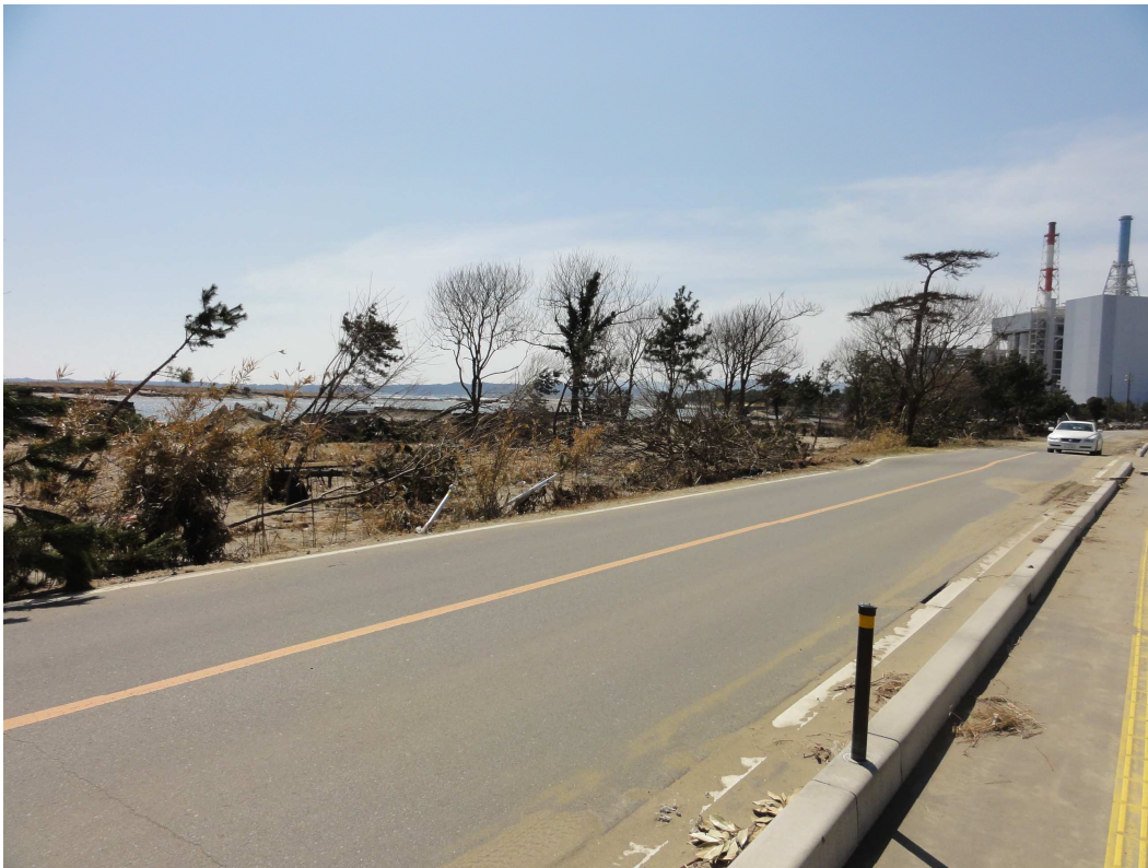
Figure 9. Fallen trees and road signs, representing the southward flow of the tsunami (March 25, 2011)
