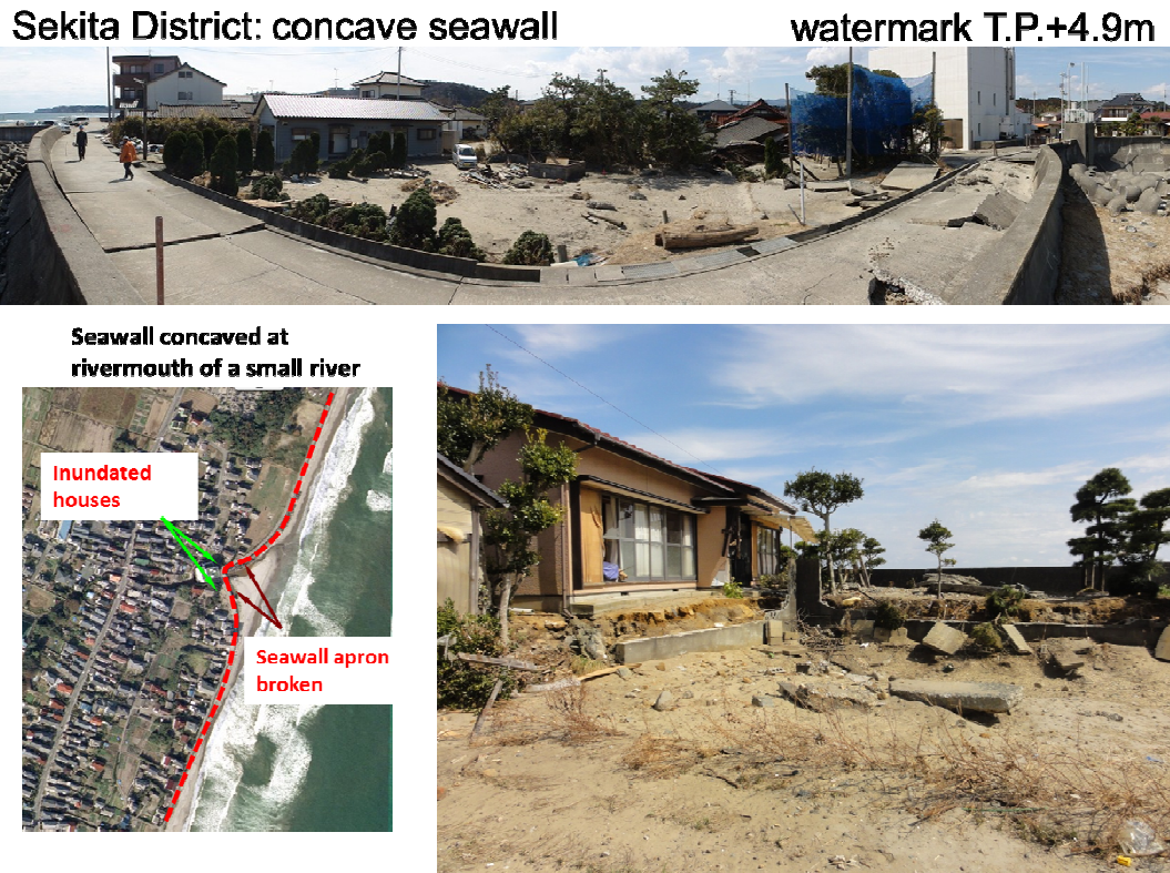
Figure 14. Damage concentrated to a concave seawall in Sekita District. (March 24, 2011)
