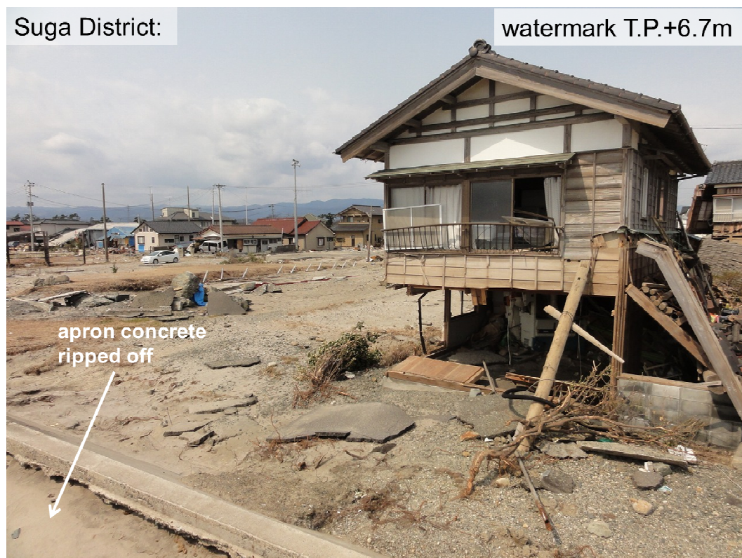
Figure 11. Broken seawall and a house in Suga District. (March 25, 2011)
