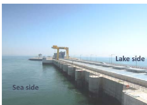
Figure 1. Sihwa tidal power plant in Korea.
