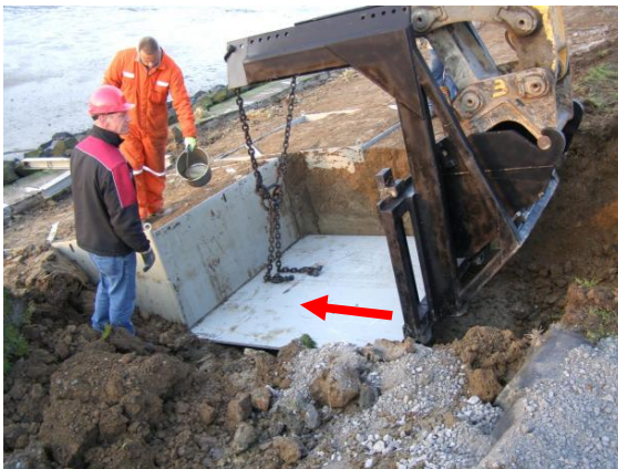
Figure 9, Pushing the steel plate underneath the clay block
