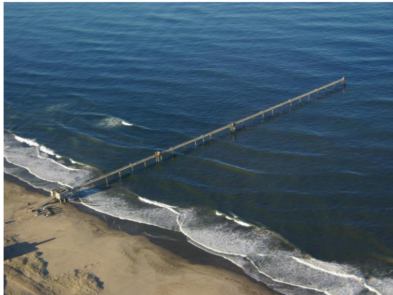
Photo 1. The pier at Hazaki Oceanographical Research Station.
