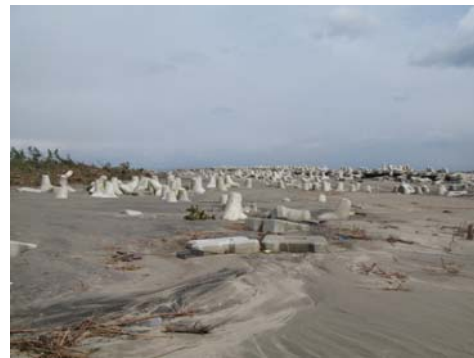
Photo 9. Scatter of the dissipation blocks behind the levee.
