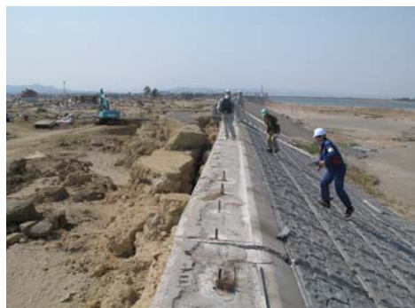
Photo 14. Three sides of the river levee.
