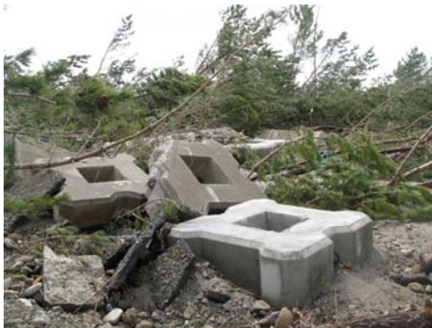
Photo 8. Scatter of the armor blocks in the woods
