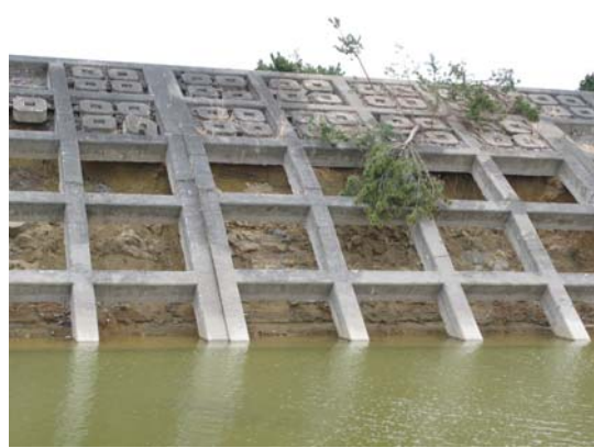
Photo 21. Landside armor blocks of the levee, and a created channel, northern Yamamoto Coast.
