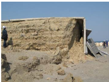
Photo 13. End section of the river levee.
