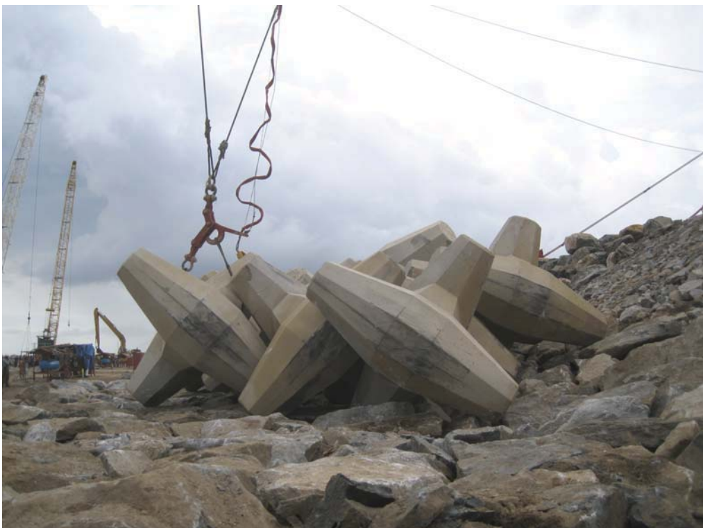
Figure 10: Toe Reinforcement – Placement of second row (Dry Trial Row 03)
