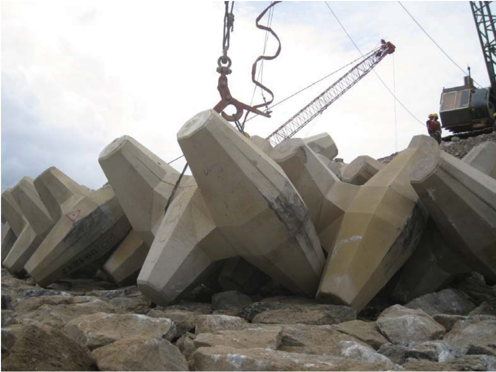
Figure 11: Toe Reinforcement – second row complete (Dry Trial Row 03)
