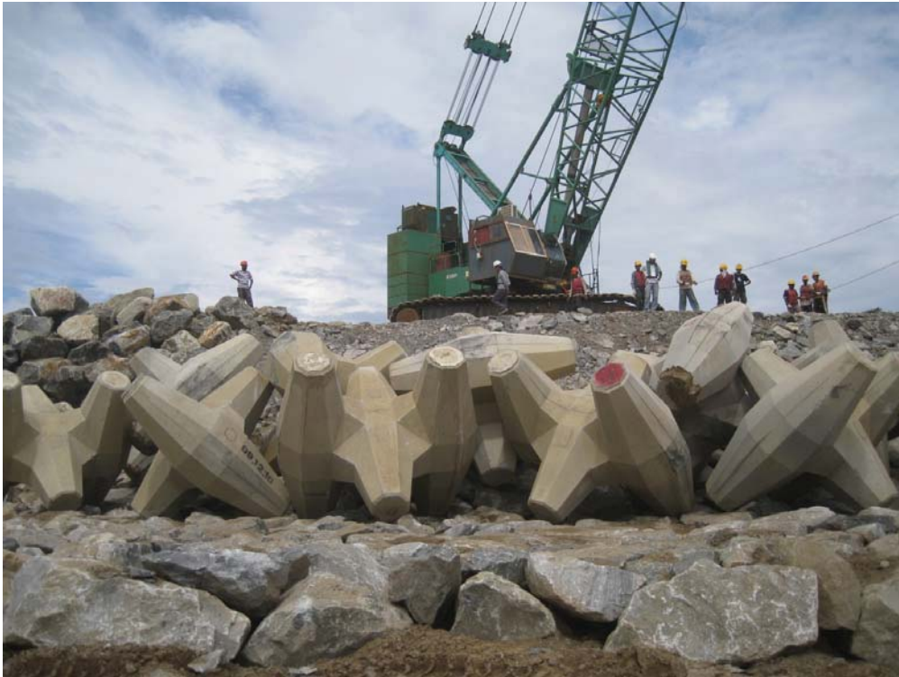
Figure 7: Start of Dry Trial – view of primary armour toe row (Row 01)
