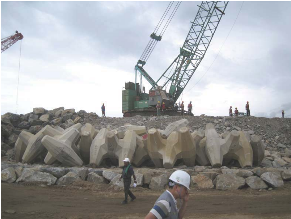
Figure 9: Toe Reinforcement – first row complete (Dry Trial Row 02)
