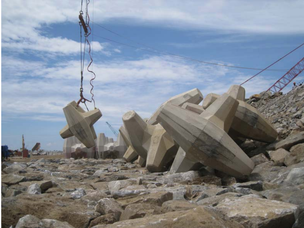
Figure 8: Toe Reinforcement – Placement of first row (Dry Trial Row 02)
