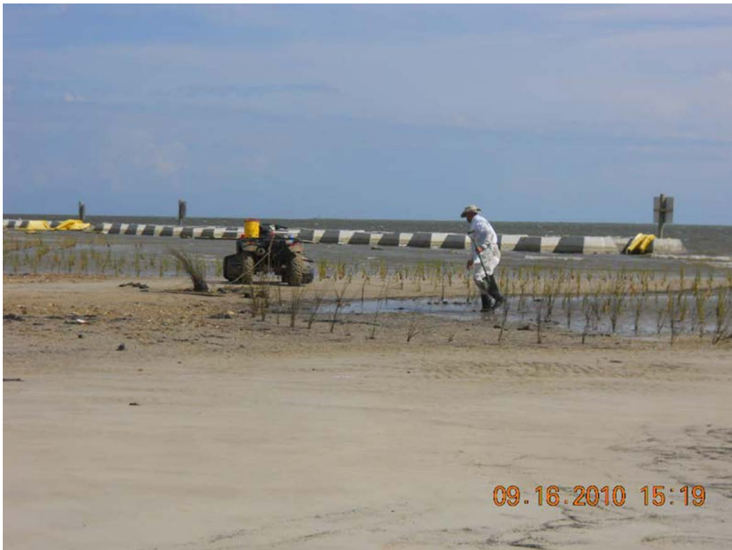
Figure 6. Planting of the S. alterniflora vegetation in the Little Bay Project by the contractor's biologist
