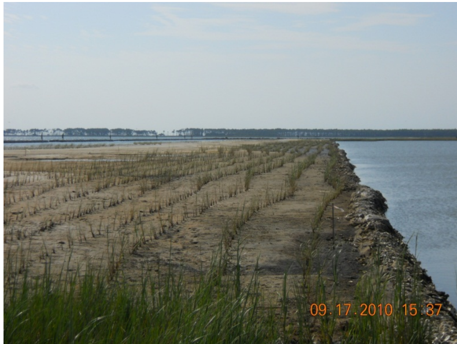
Figure 7. The bagged oyster shell breakwater used on the north side of the peninsula restoration area to hold the fill out of Little Bay.
