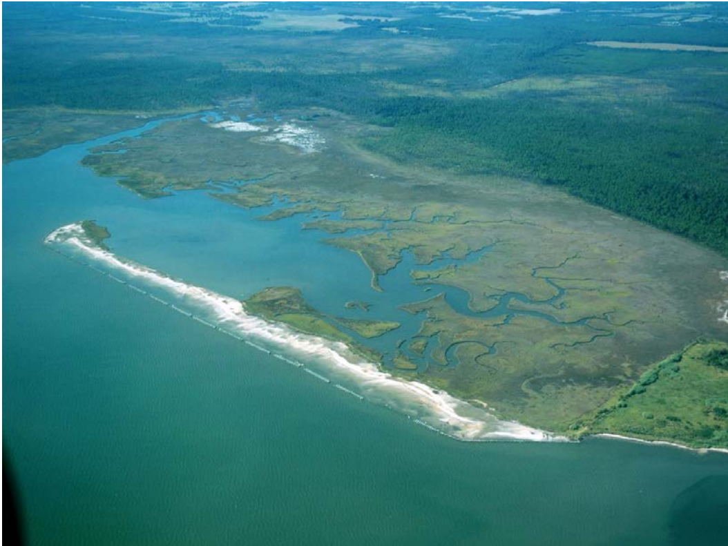
Figure 5. The Little Bay Project immediately after construction was completed. Note the breakwater structure including the gaps, the new sand, and the restoration of the peninsula defining Little Bay.
